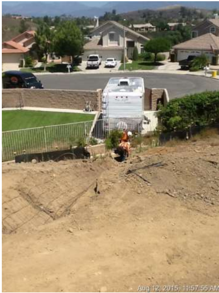
Figure 5: Drainage devices installed between VC #5 and VC #6, 500 kV Underground.
