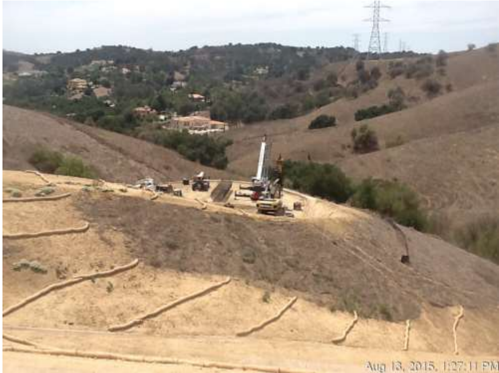
Figure 1: Foundation drilling at Tower M60-T1X at the WTS, 500 kV Underground.
