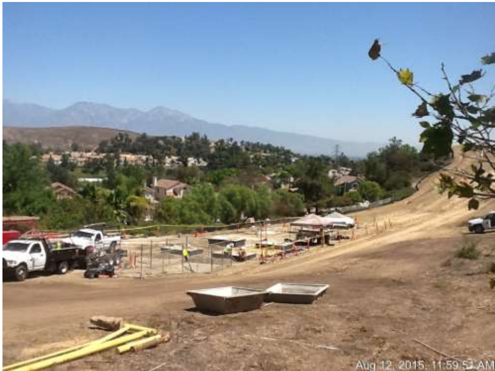
Figure 2: Concrete apron installation activities at VC #7, 500 kV Underground.
