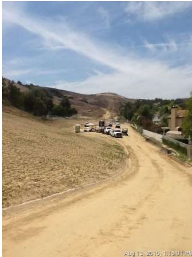
Figure 4: Clean, proof and mandrel activities occurred at VC #5, 500 kV Underground.
