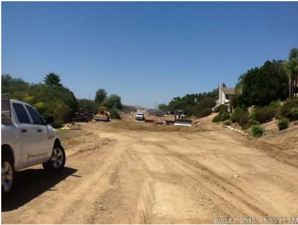
Figure 5: Grading activities at VC #10, 500 kV Underground.
