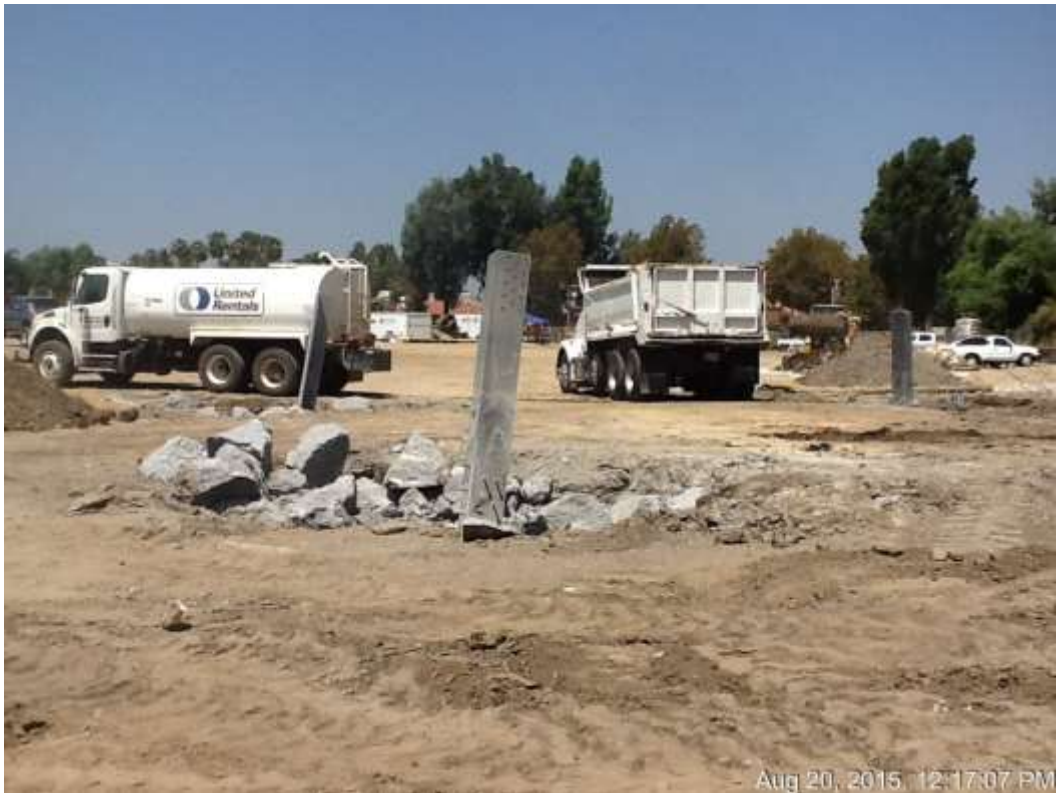
Figure 4: Foundation demolition at Construct M64-T1 at the ETS, 500 kV Underground.
