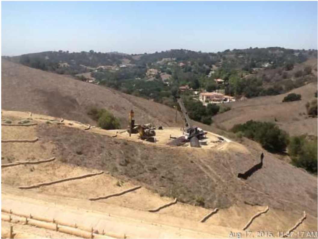
Figure 3: Foundation installation activity at Construct M60-T1X at the WTS, 500 kV Underground.
