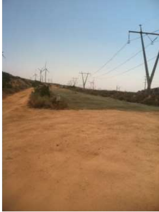
Figure 1: Hydroseed application at Ground Rod 15 disturbance area, Segment 3B AC Mitigation.
