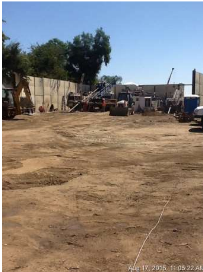
Figure 6: HDD activity at VC #12, 500 kV Underground.
