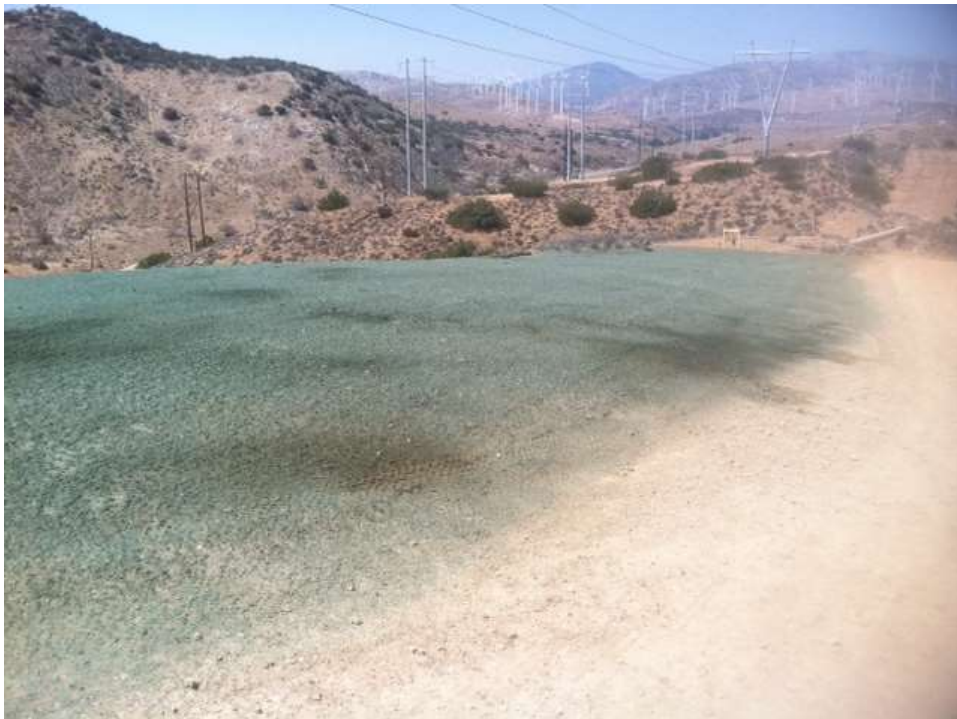
Figure 2: Hydroseed application at span burial site, Segment 3B AC Mitigation.
