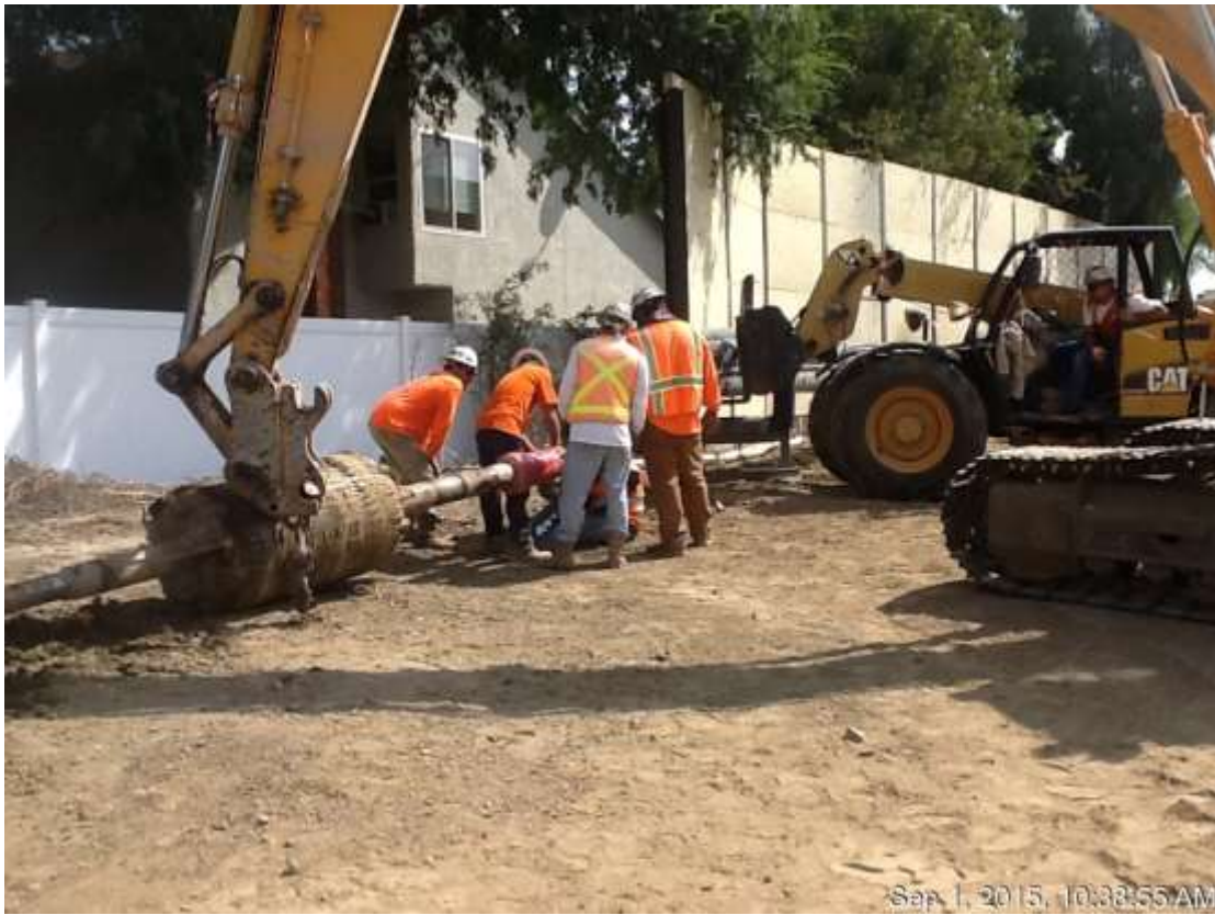
Figure 3: Conduit pulling preparation at HDD C1-S2, 500 kV Underground.
