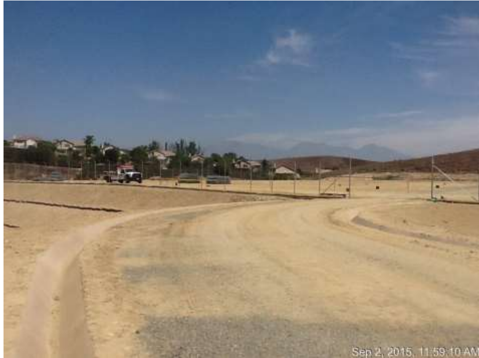
Figure 1: Temporary fence installation activities at the WTS, 500 kV Underground.
