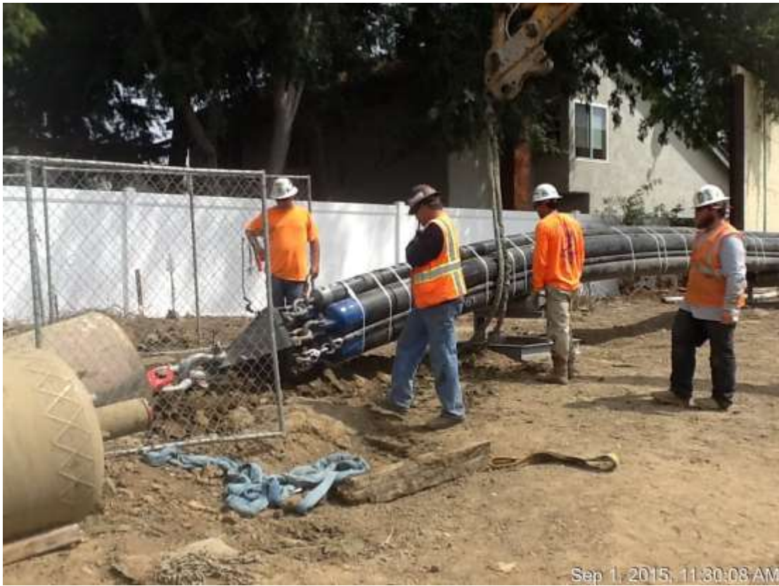
Figure 5: Conduit pulling activities at HDD C1-S2, 500 kV Underground.
