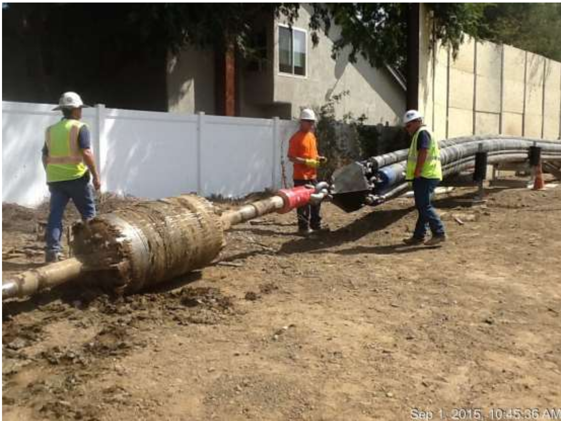
Figure 4: Conduit pulling activities at HDD C1-S2, 500 kV Underground.
