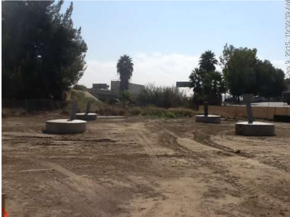
Figure 1: Transition structure foundation installation occurred at the ETS, 500 kV Underground.
