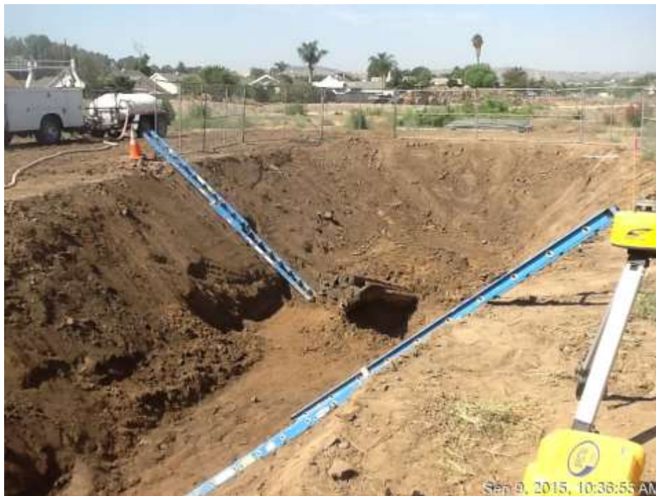
Figure4: Trenching at short bore HDD toward VC #14, 500 kV Underground.
