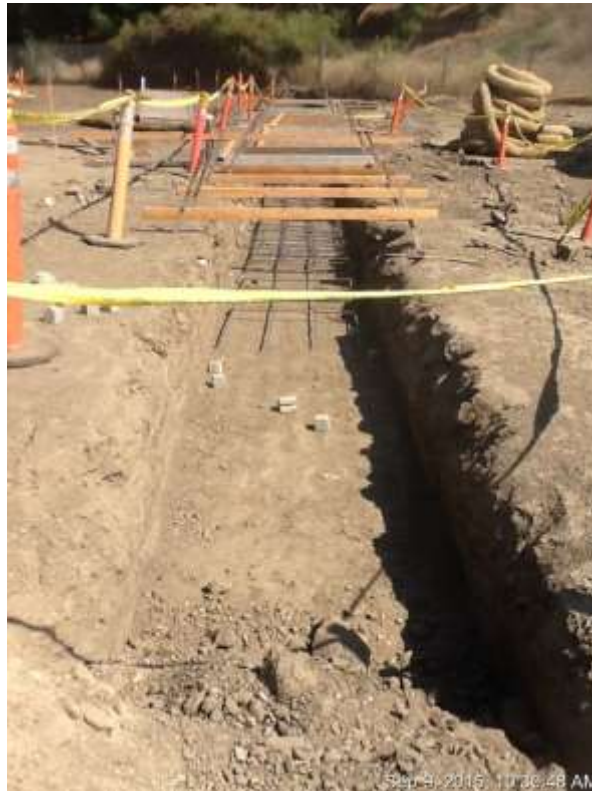
Figure 2: Perimeter wall installation occurred at the ETS, 500 kV Underground.
