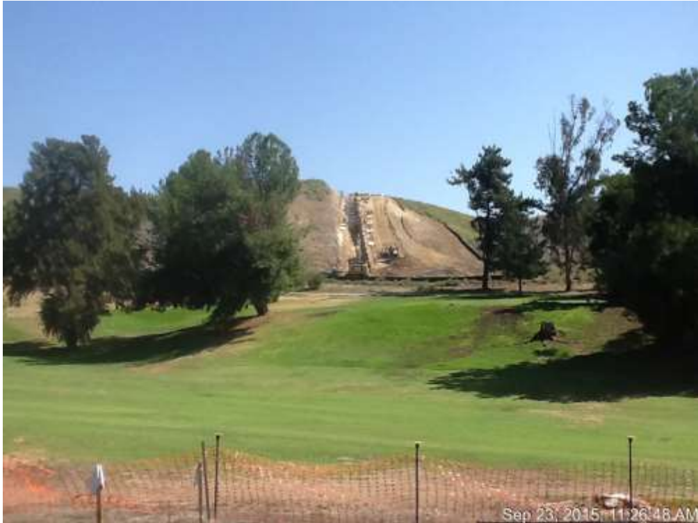
Figure 1: Trench excavation between RV#2 toward the Golf Course, 500 kV Underground.
