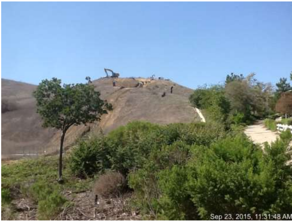
Figure 2: Grading activities between VC #4 and RV #4, 500 kV Underground.
