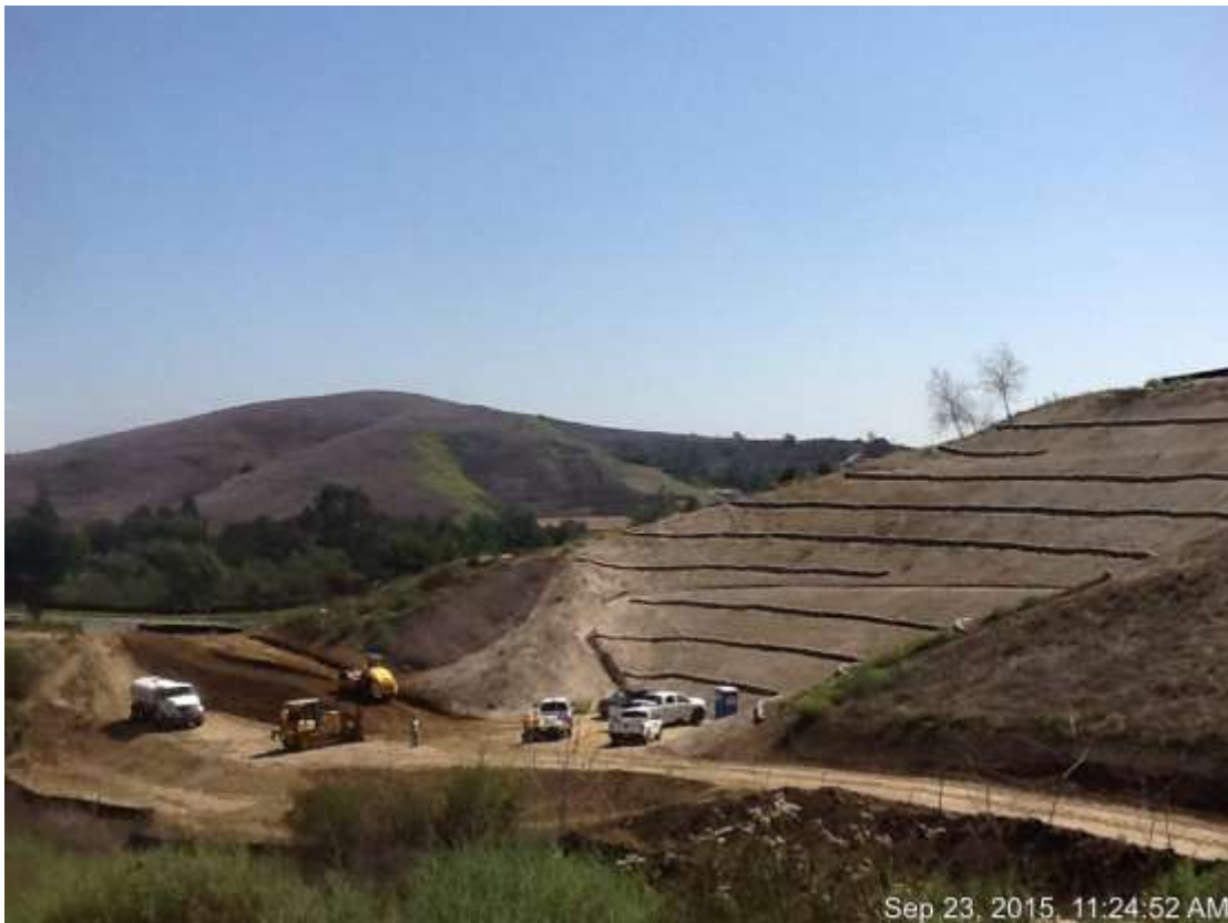
Figure4: RV #1 pad preparation for vault delivery, 500 kV Underground.
