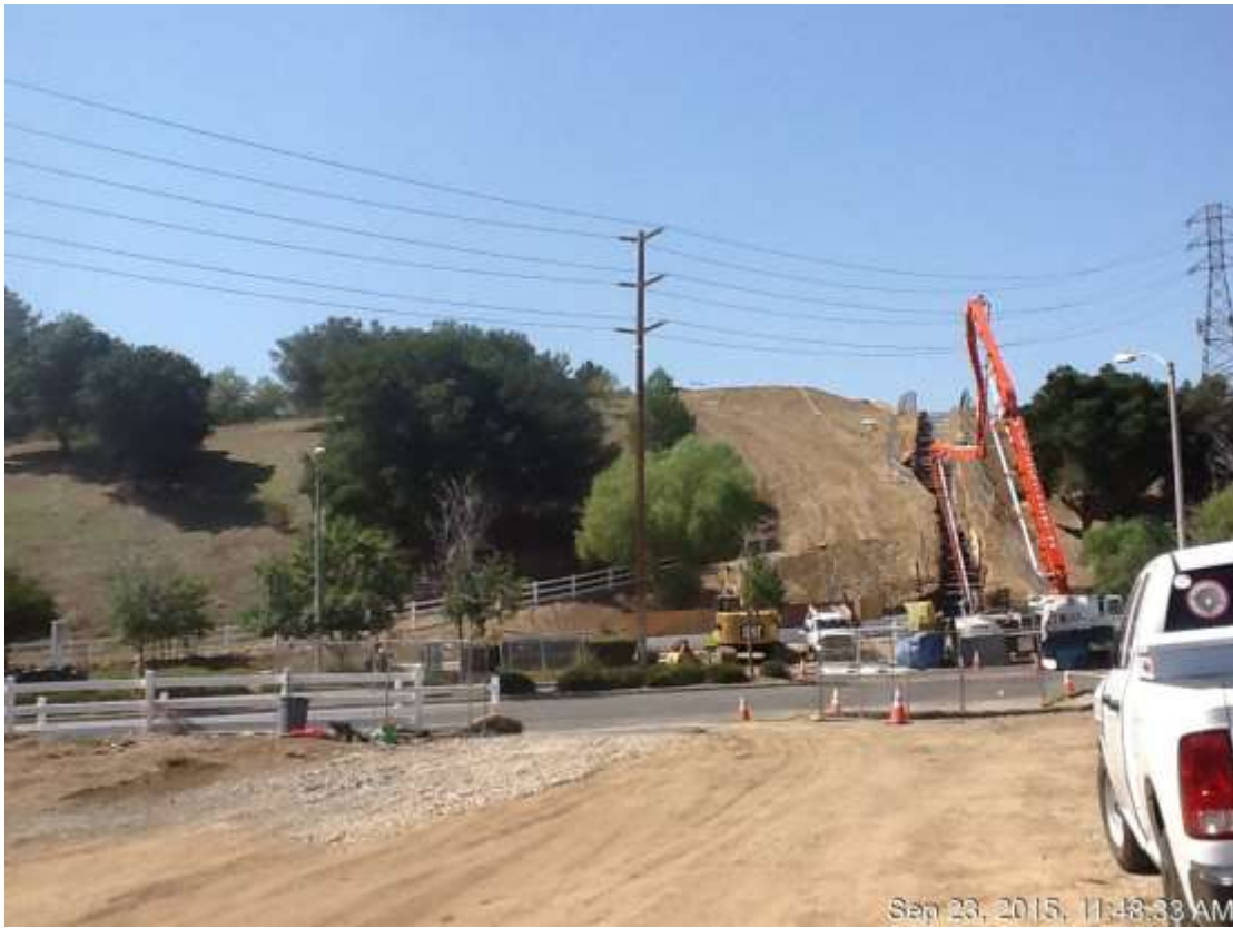
Figure 3: Concrete backfill between VC #8 and Chino Hills Parkway, 500 kV Underground.
