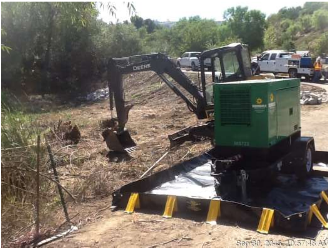
Figure 3: Vegetation removal from stream diversion area near VC #2, 500 kV Underground.
