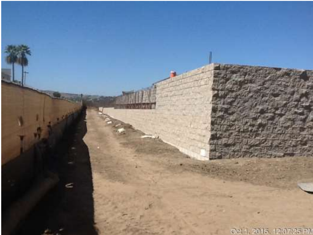
Figure 2: ETS wall construction, 500 kV Underground.
