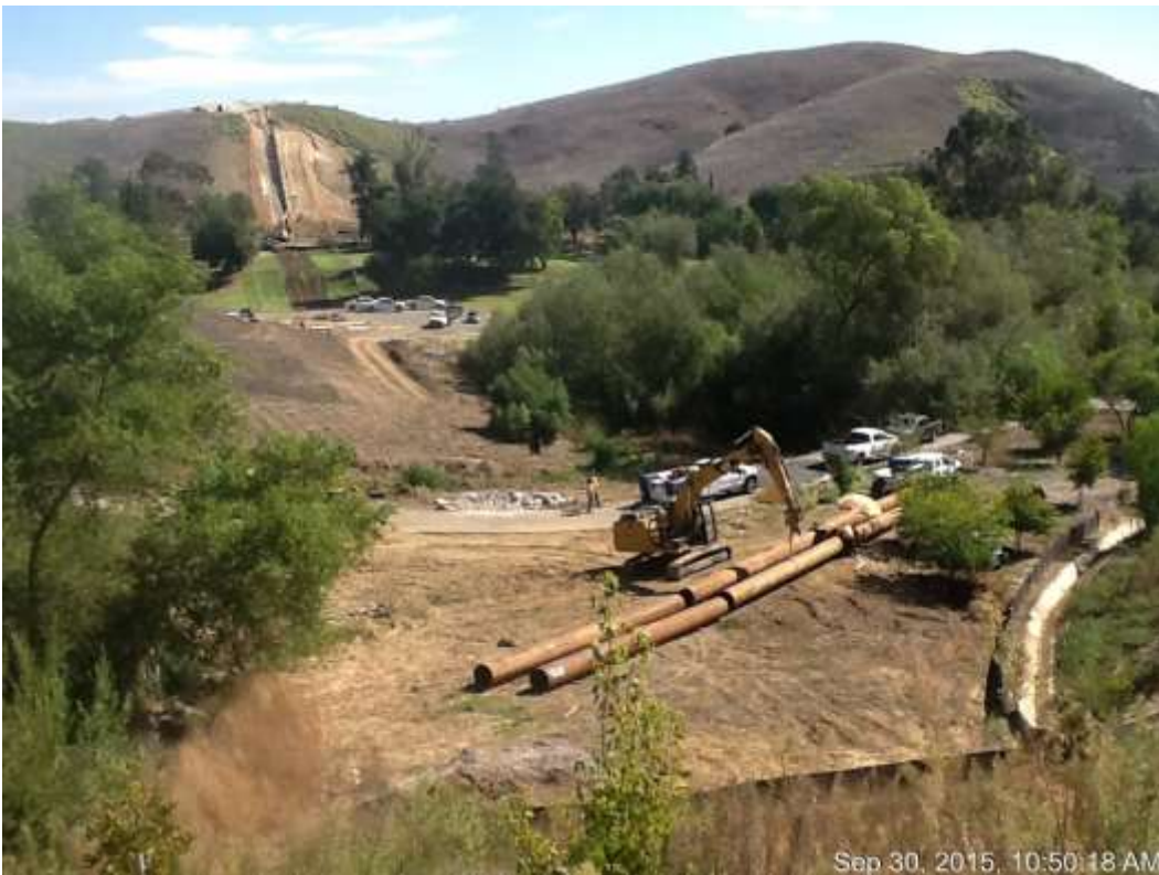
Figure 4: Diversion pipe fabrication at stream diversion area near VC #2, 500 kV Underground.
