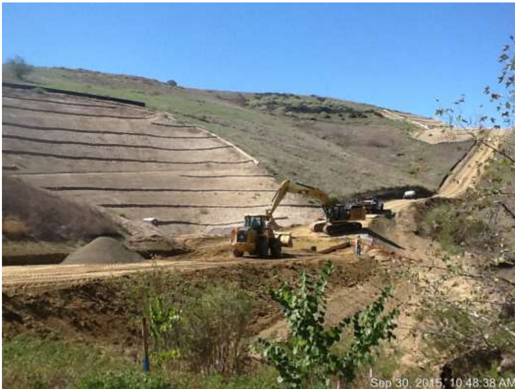
Figure 5: VC #1 excavation for vault placement, 500 kV Underground.
