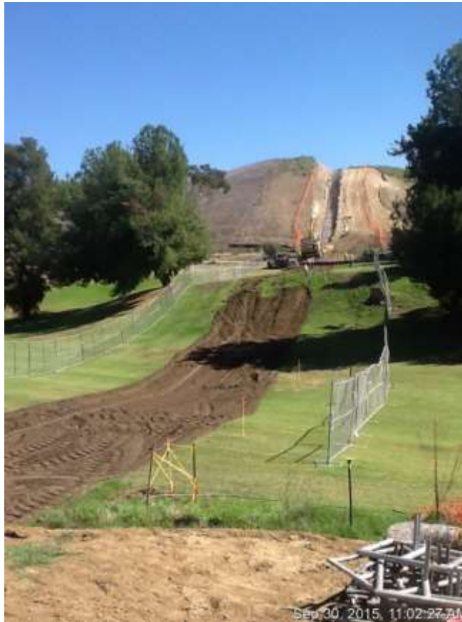
Figure 6: Vegetation removal of trenchline between RV #2 and VC #2, 500 kV Underground.
