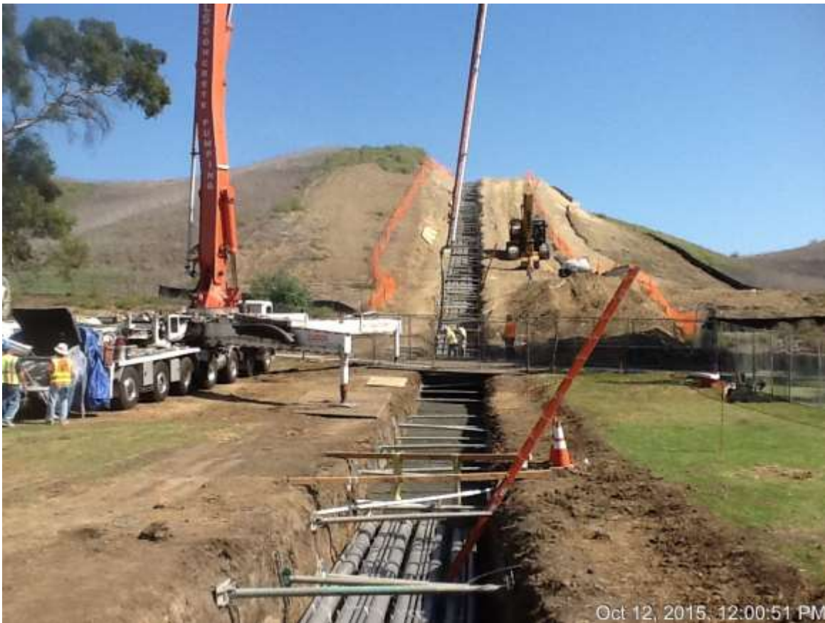
Figure 5: Conduit installation between RV#2 and VC #2 via golf course, 500 kV Underground.
