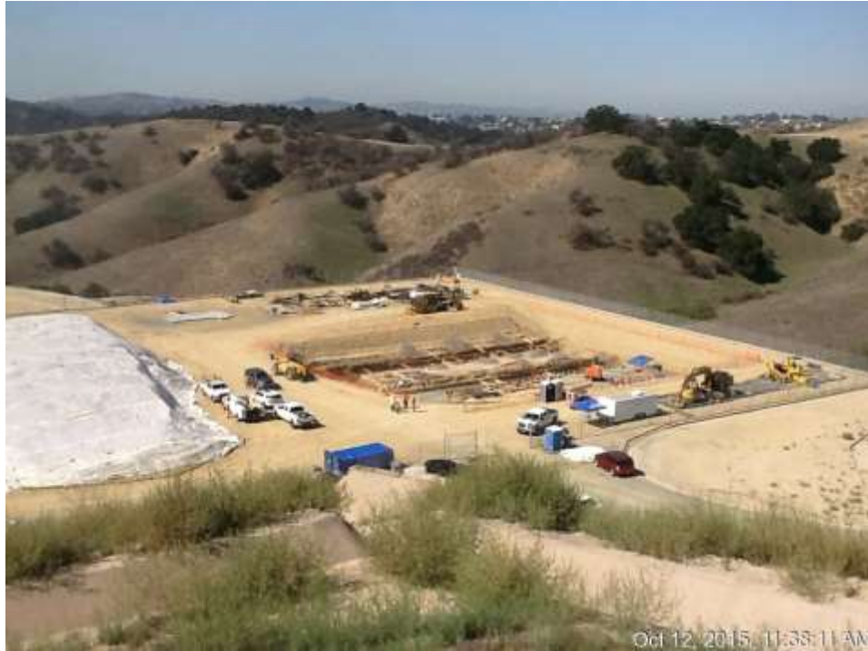
Figure 1: WTS foundation activities for the MEER building, 500 kV Underground.
