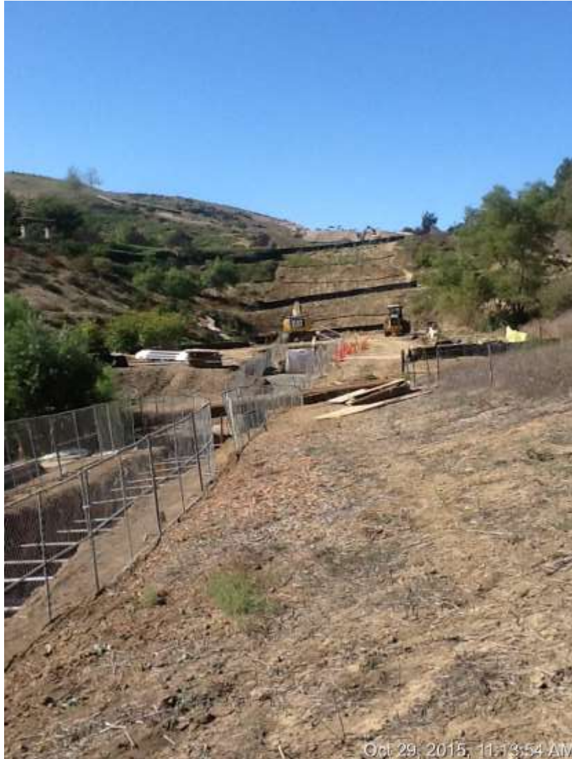
Figure 1: Stream diversion location between VC #2 and VC #3, 500 kV Underground.
