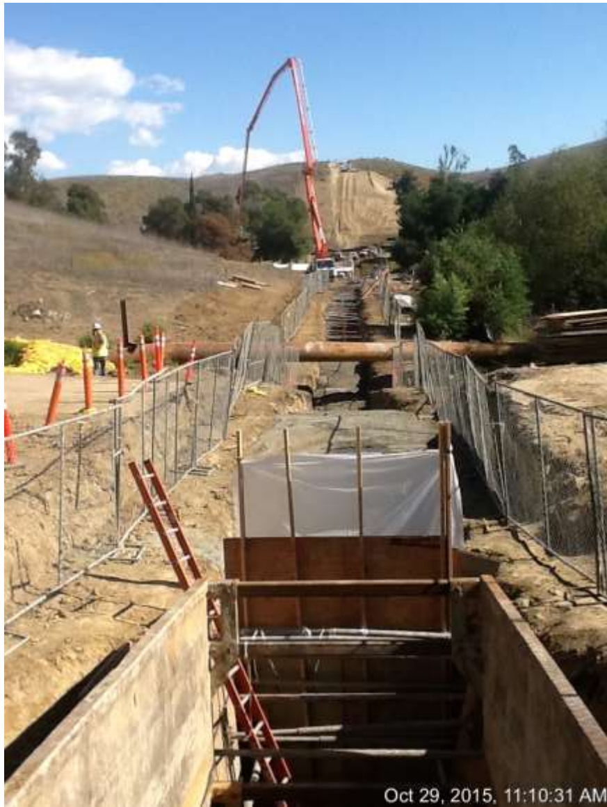
Figure 3: Backfilling operations near the stream diversion near VC #2, 500 kV Underground.
