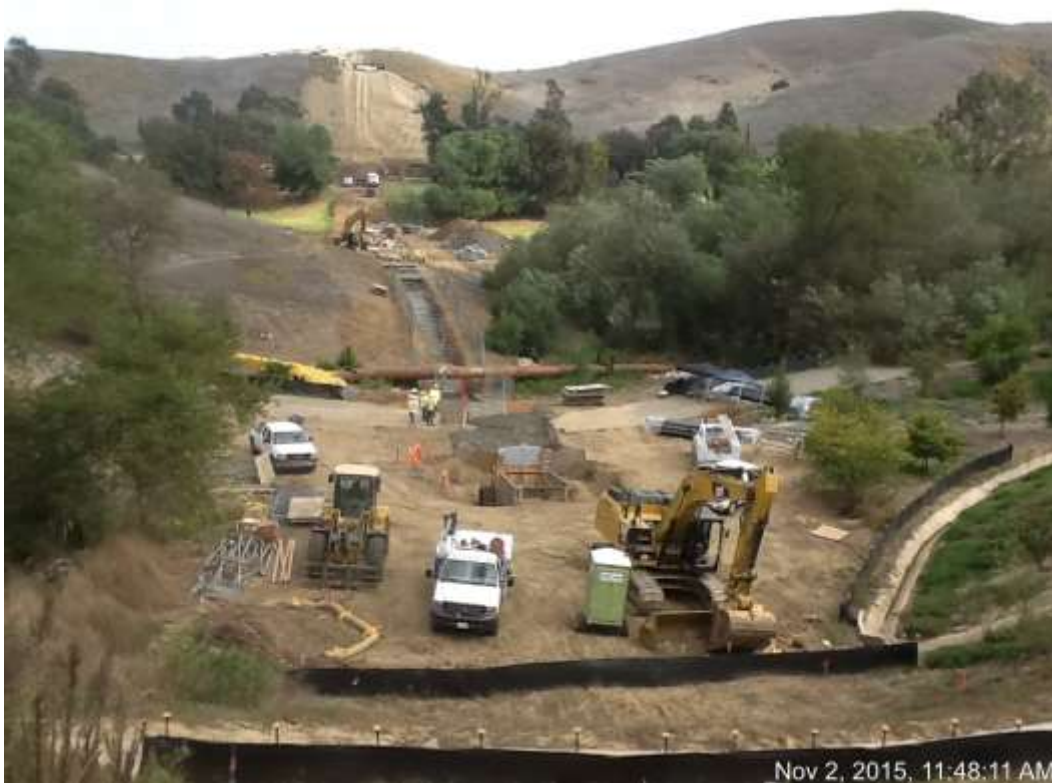
Figure 4: Backfilling operations near the stream diversion near VC #2, 500 kV Underground.
