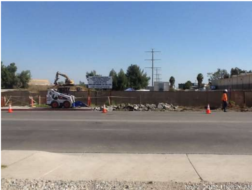
Figure 2: Driveway demolition at the ETS, 500 kV Underground.
