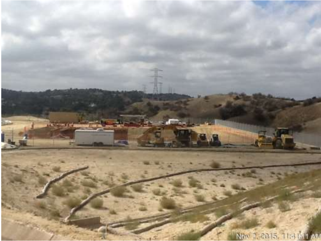
Figure 1: Construction activities at the WTS, 500 kV Underground.
