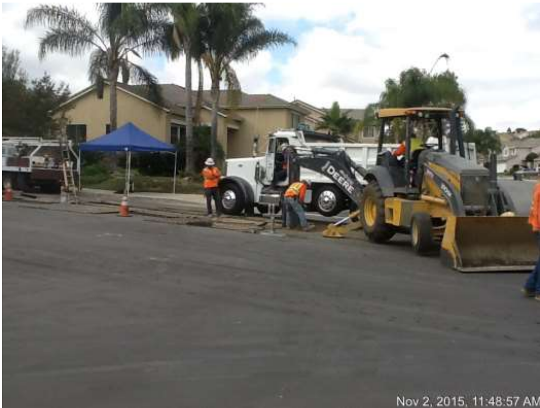
Figure 3: Telecom trenching and conduit installation along Eucalyptus Avenue, 500 kV Underground.
