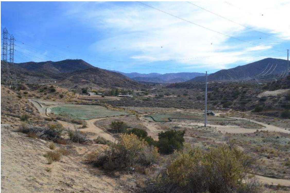
Figure 2: Construction disturbance areas were hydroseeded near the Vincent Substation, Segment 11C.
