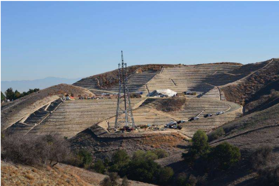
Figure 6: Assembly of Tower M60-T1X at the WTS, 500 kV Underground.
