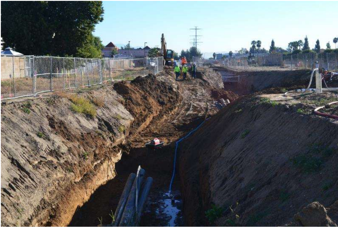
Figure 5: Trench dewatering was conducted at the VC #14 tie-in location, 500 kV Underground.
