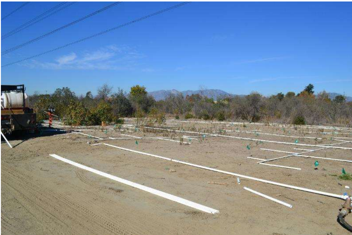
Figure 4: Irrigation system installation occurred at Tower M41-T5 in Whittier Narrows, Segment 8.
