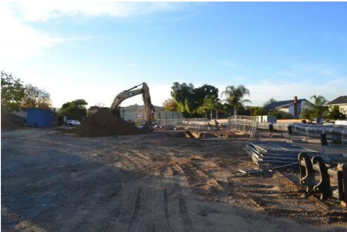
Figure 2: Excavation for cable trench tie-in at VC #12, 500 kV Underground.
