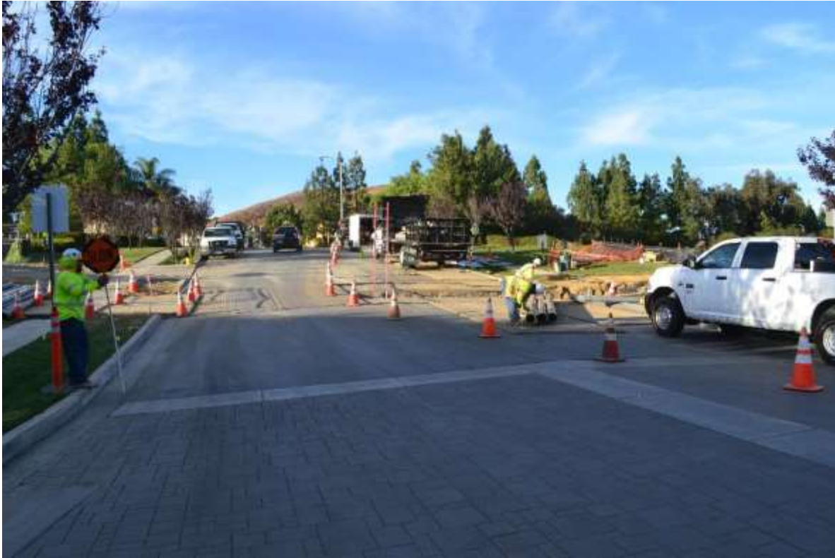
Figure 1: Cable trenching across Canon Lane in Chino Hills, 500 kV Underground.
