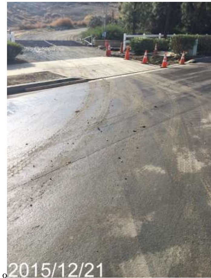
Figure 2: Track out observed on Eucalyptus Avenue near the WTS entrance, photo courtesy of FRED.
