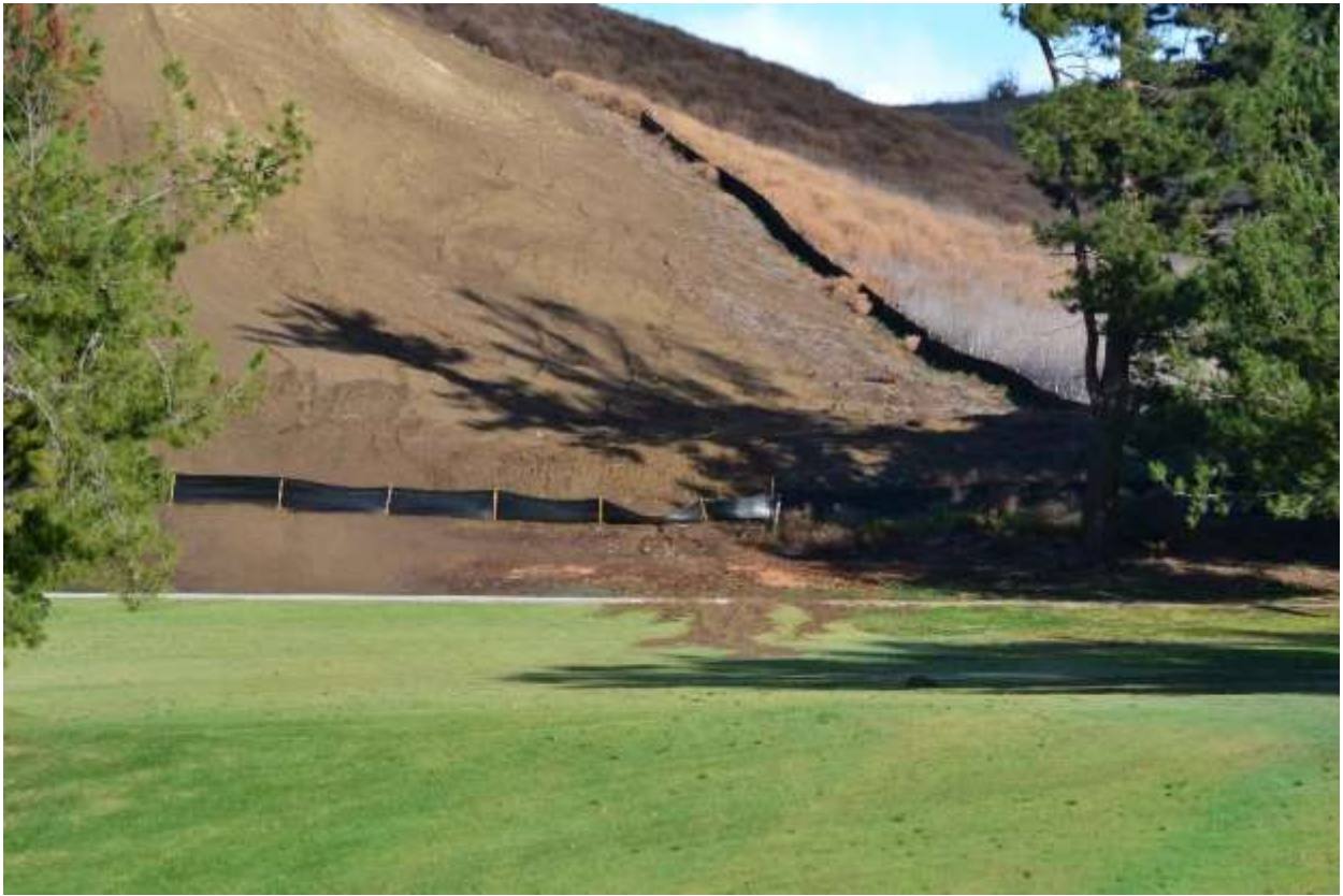
Figure 3: Sediment discharge incident at the golf course near VC #2, Chino Hills Underground.
