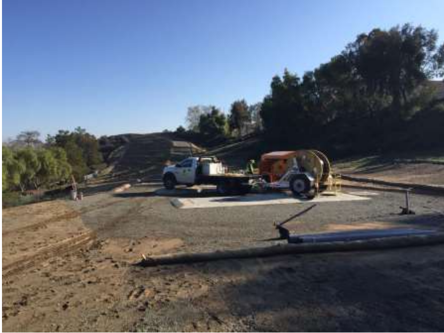
Figure 1: Underground cable installation between VC #5 and VC #7, Chino Hills Underground.
