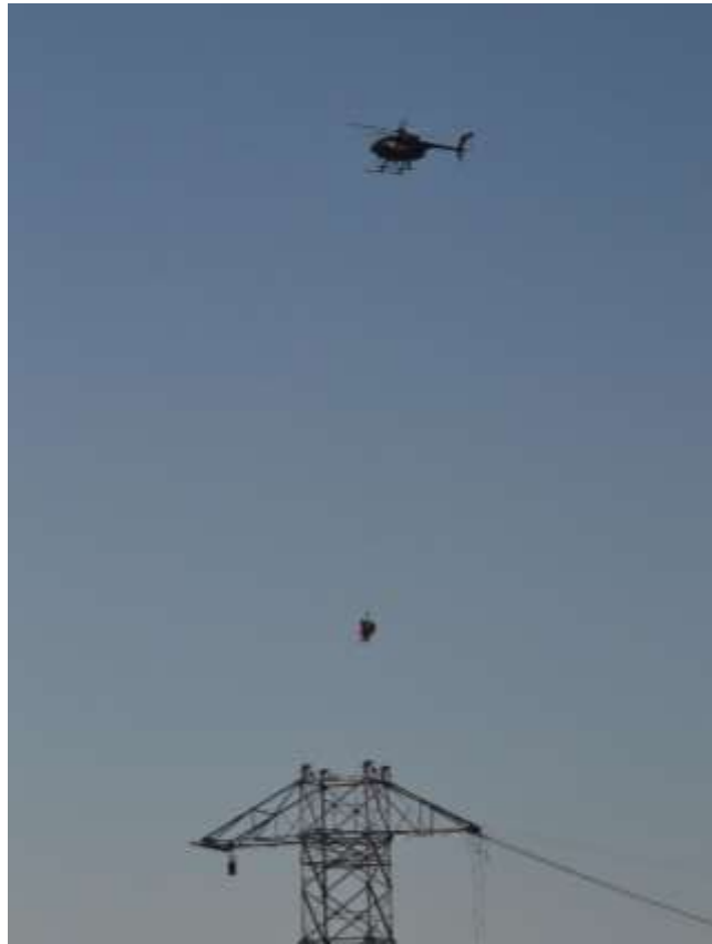
Figure 2: Helicopter operations and conductor installation west of the WTS.
