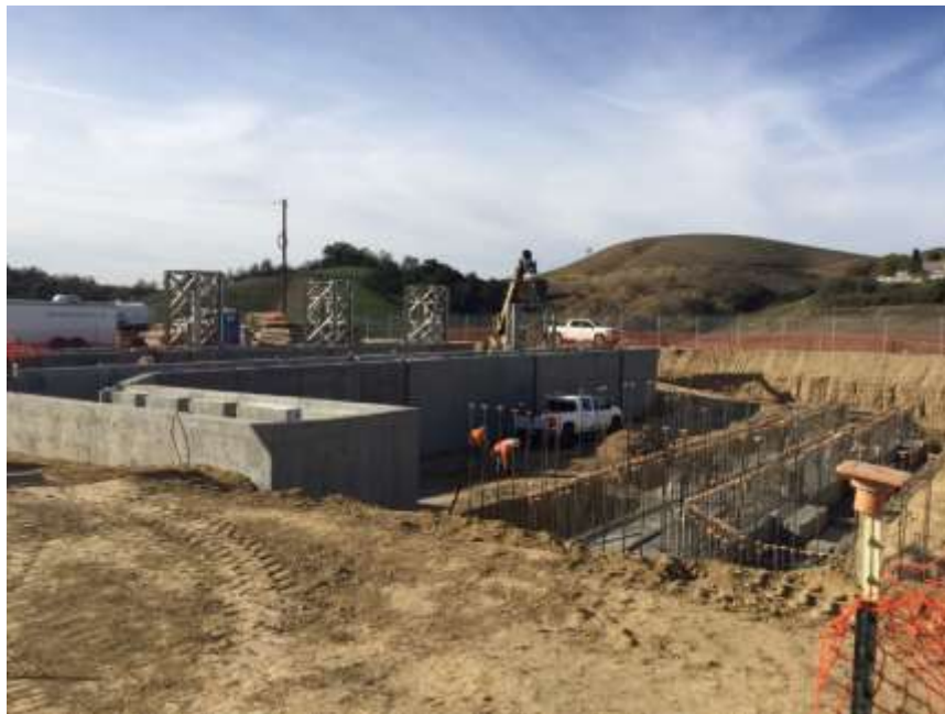
Figure 4: Trench work and wall installation continue at the Western Transition Station.
