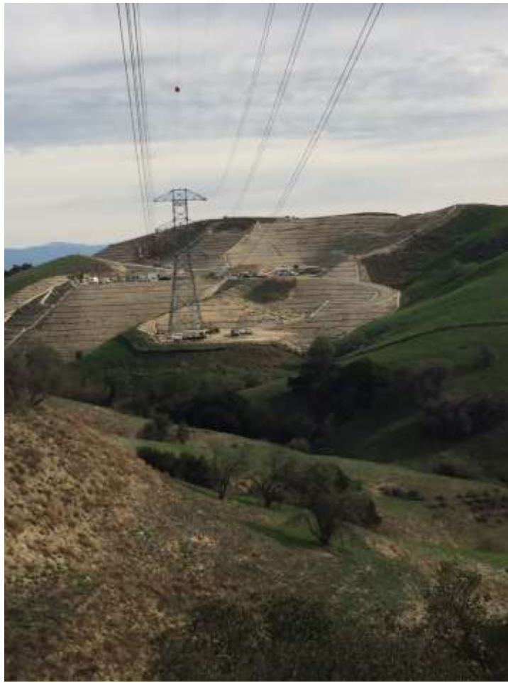
Figure 3: Conductor installation was completed to Tower M60-T1 near the WTS.
