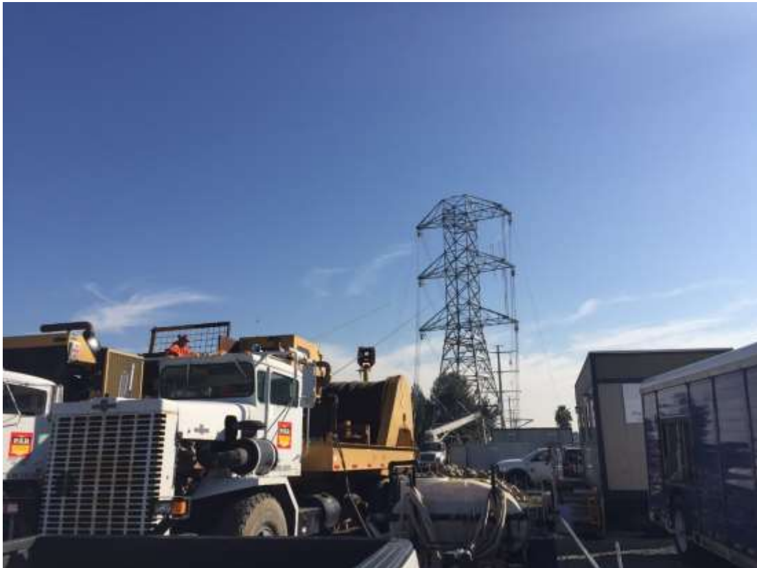
Figure 4: Conductor stringing to Tower M64-T1 at the ETS, 500 kV Underground.
