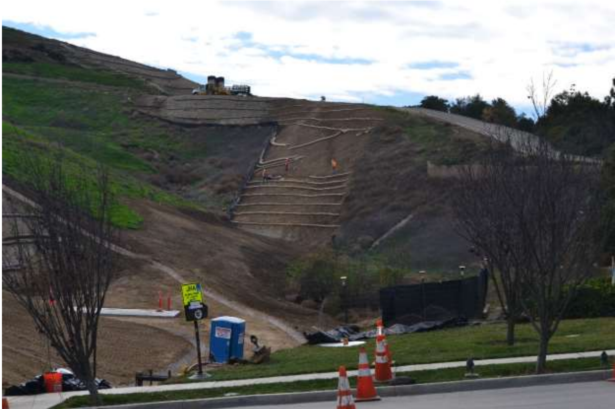
Figure 1: Permanent BMP installation along the 500 kV Underground right-of-way near VC #1.
