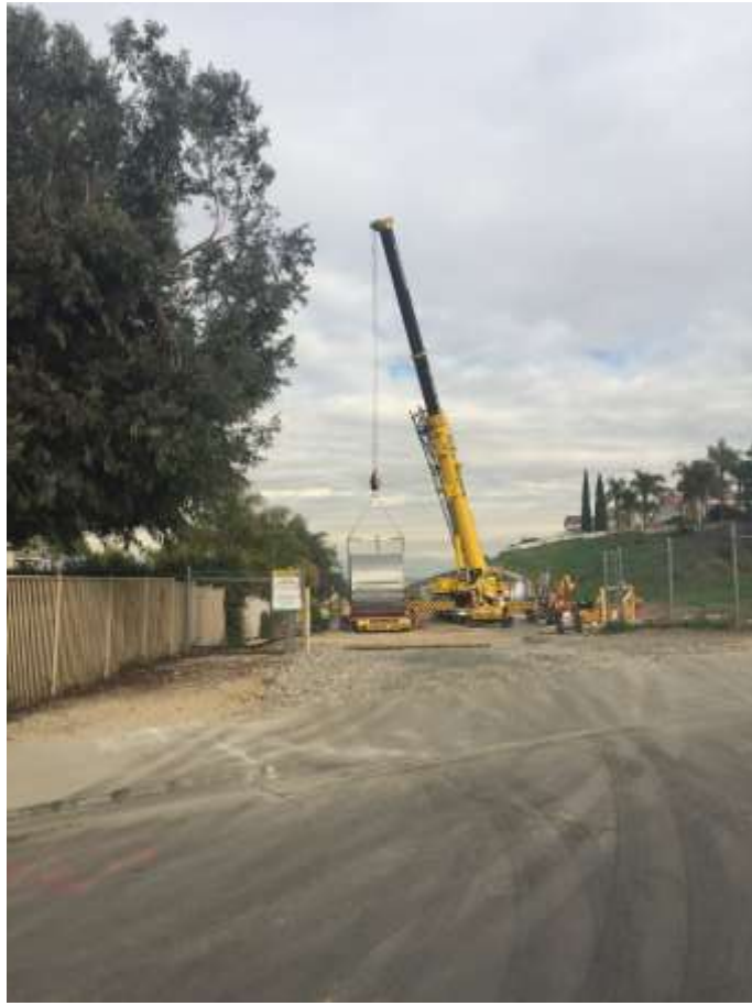
Figure 3: Cable delivery to VC #5, 500 kV Underground.
