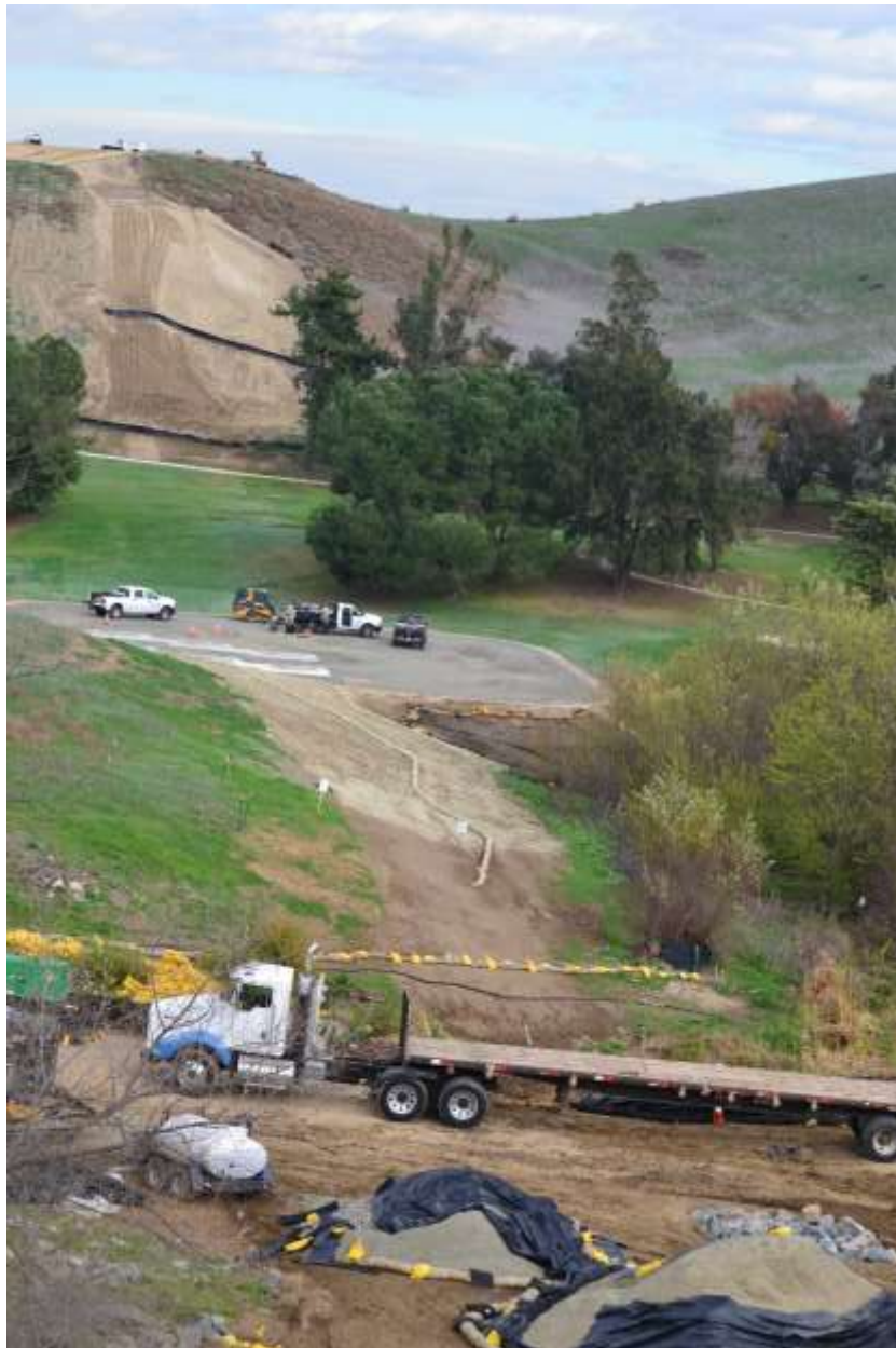
Figure 2: Crews removed the stream diversion pipe near VC #2.
