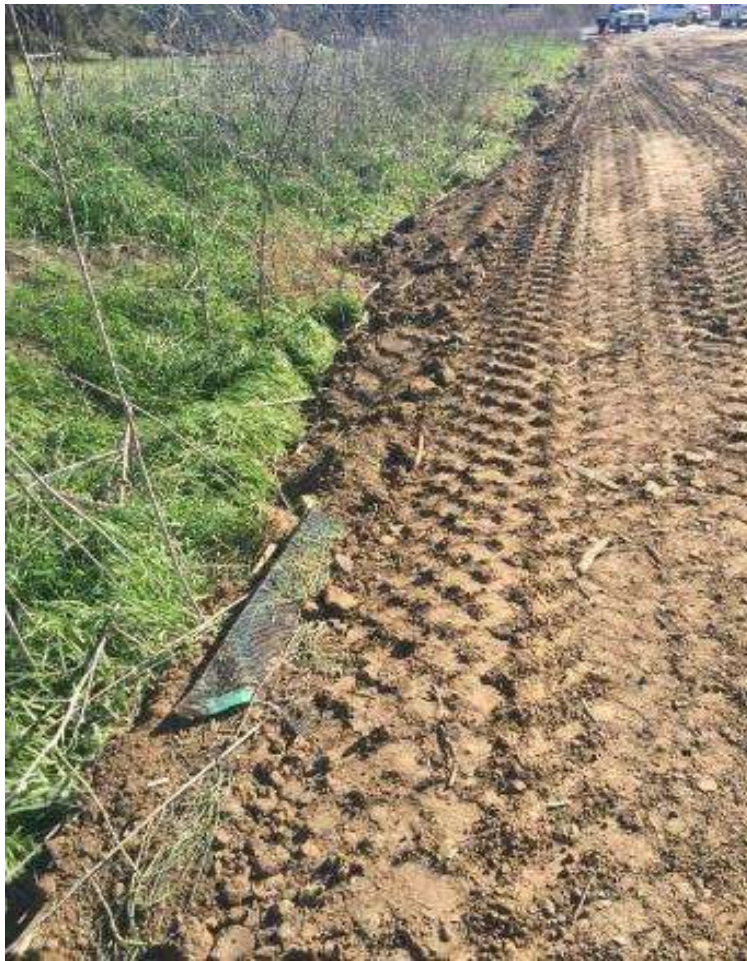
Figure 7: BMPs were buried along the access road to VC #2, 500 kV Underground.
