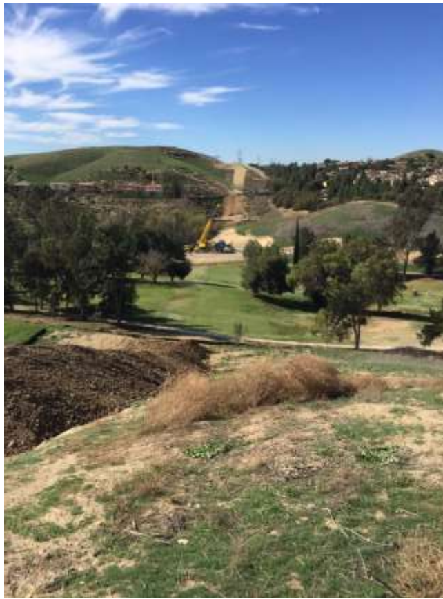
Figure 5: Cable installation between VC #2 and VC #4, 500 kV Underground.
