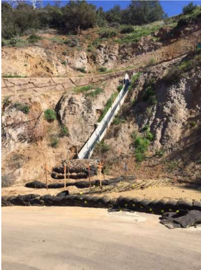
Figure 1: BMP installation and maintenance occurred at Tower M27-T3, Segment 7.
