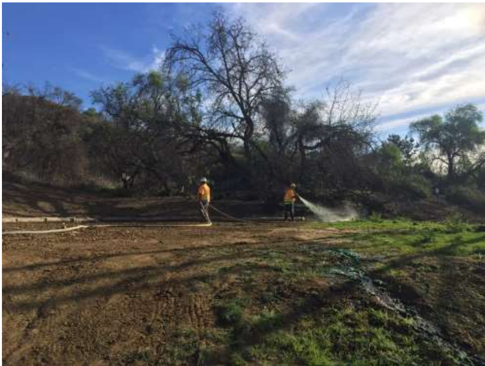
Figure 3: Hydroseeding of temporarily disturbed work areas, Segment 8 Phase 4.
