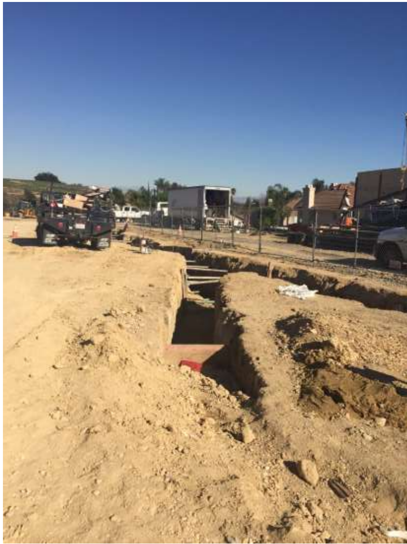
Figure 4: Tie ins continued at VC #11.
