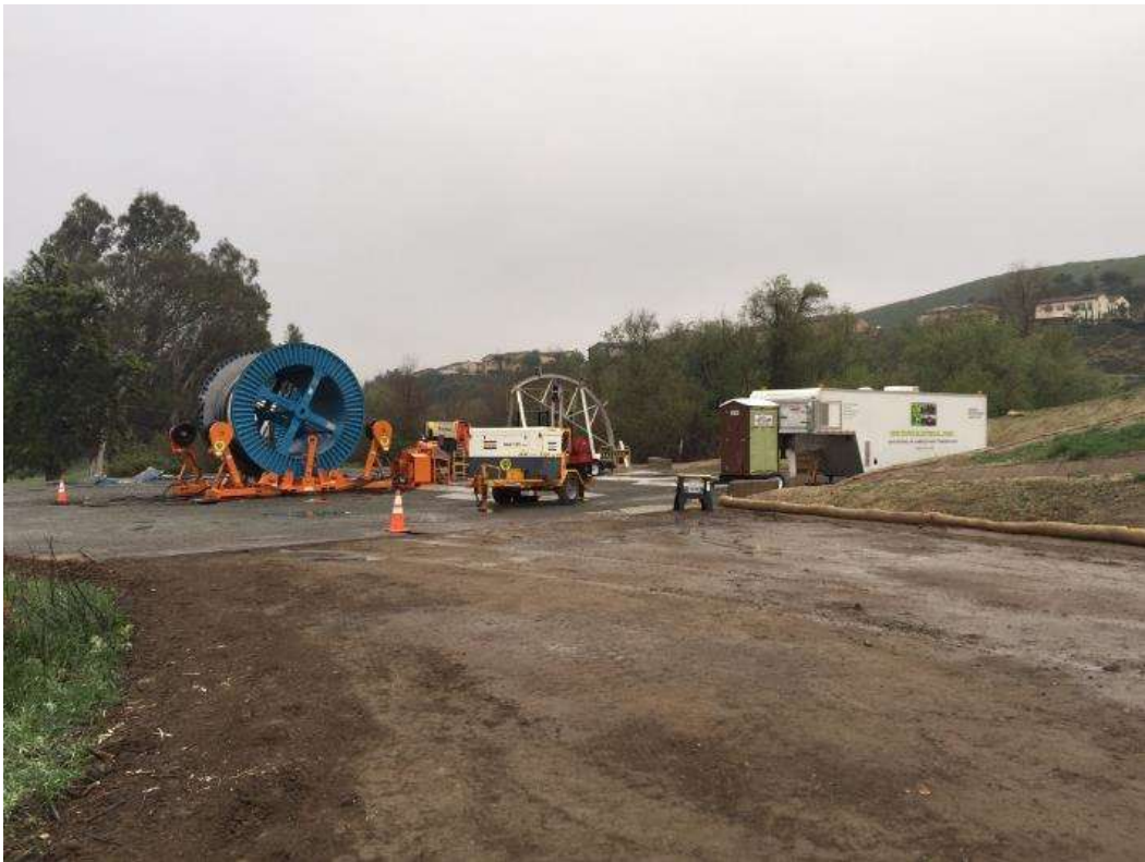
Figure 3: Cable pulling operations at VC #2, 500 kV Underground.
