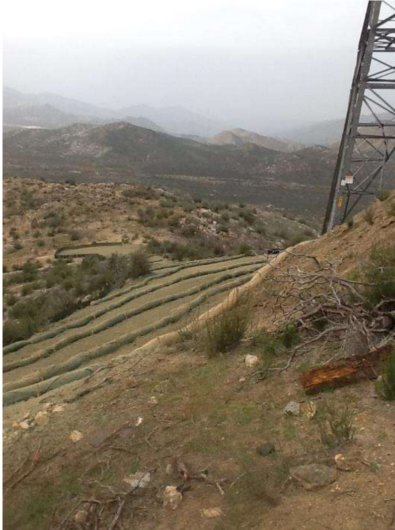
Figure 1: Restoration of graded roadway at Tower 18, Segment 11.
