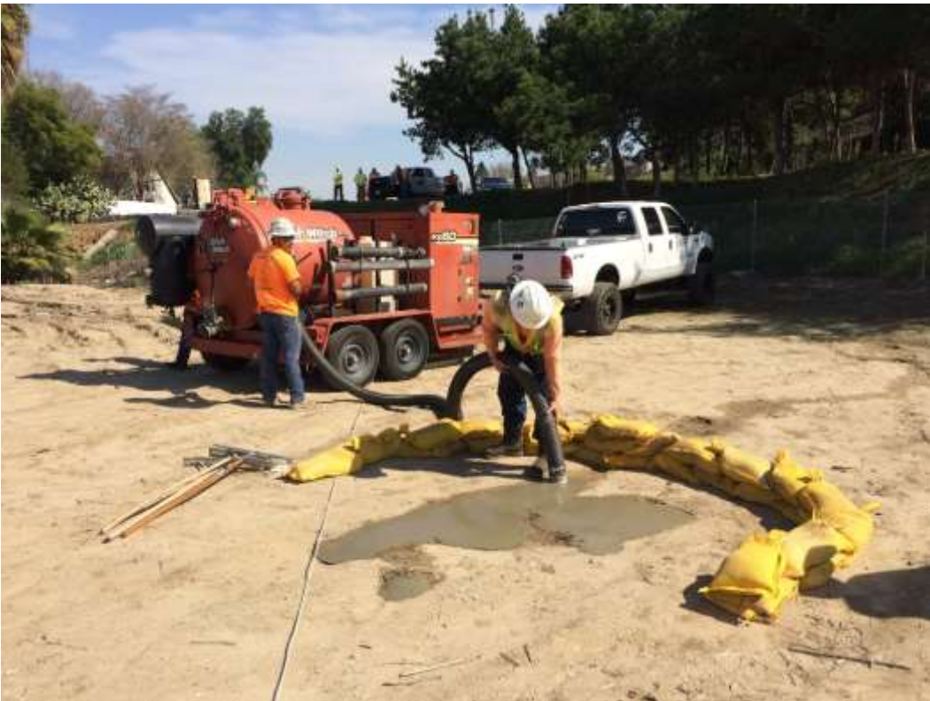
Figure 4: Frac-out clean-up near VC #12, 500 kV Underground (Photo courtesy of SCE).
