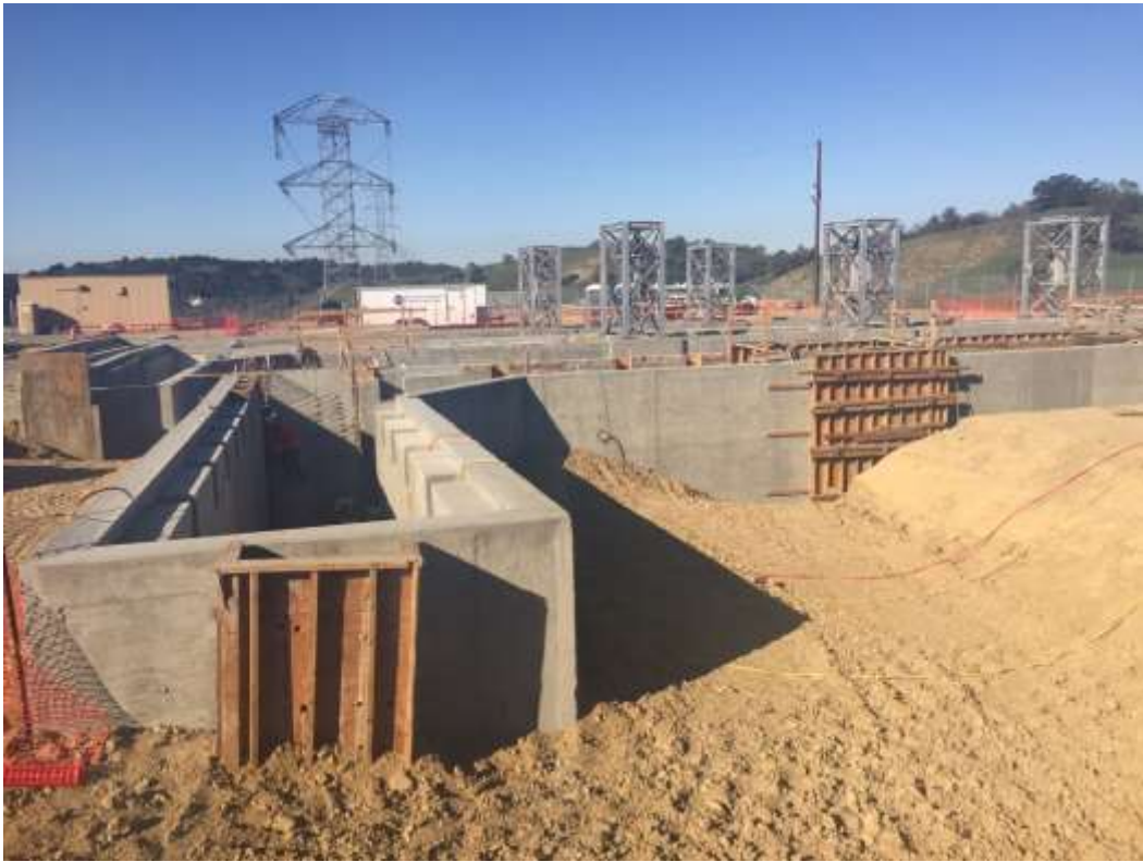
Figure 3: Cable trench construction at the Western Transition Station, 500 kV Underground.
