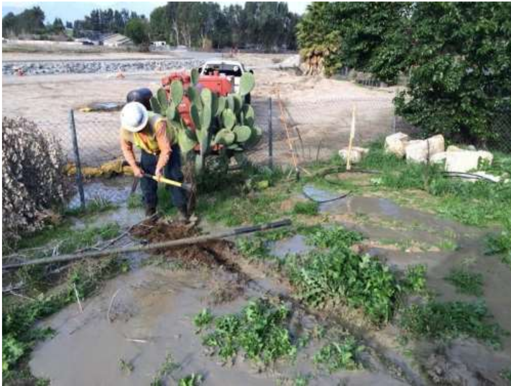
Figure 5: Frac-out clean-up near VC #12, 500 kV Underground (Photo courtesy of SCE).
