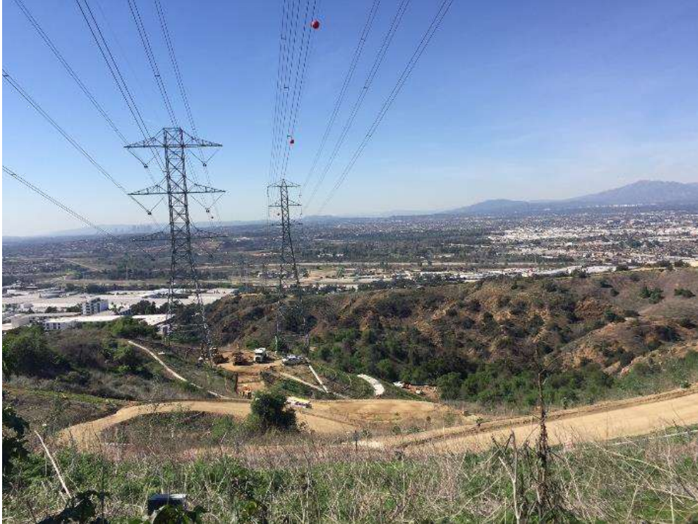
Figure 1: Grading activities continue at Tower M43-T3, Segment 8 Phase 4.
