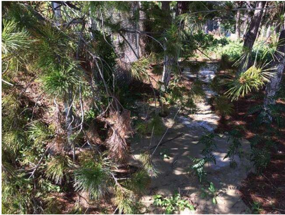
Figure 7: Frac-out near VC #12 through buffer for nesting bird, 500 kV Underground (Photo courtesy of SCE).
