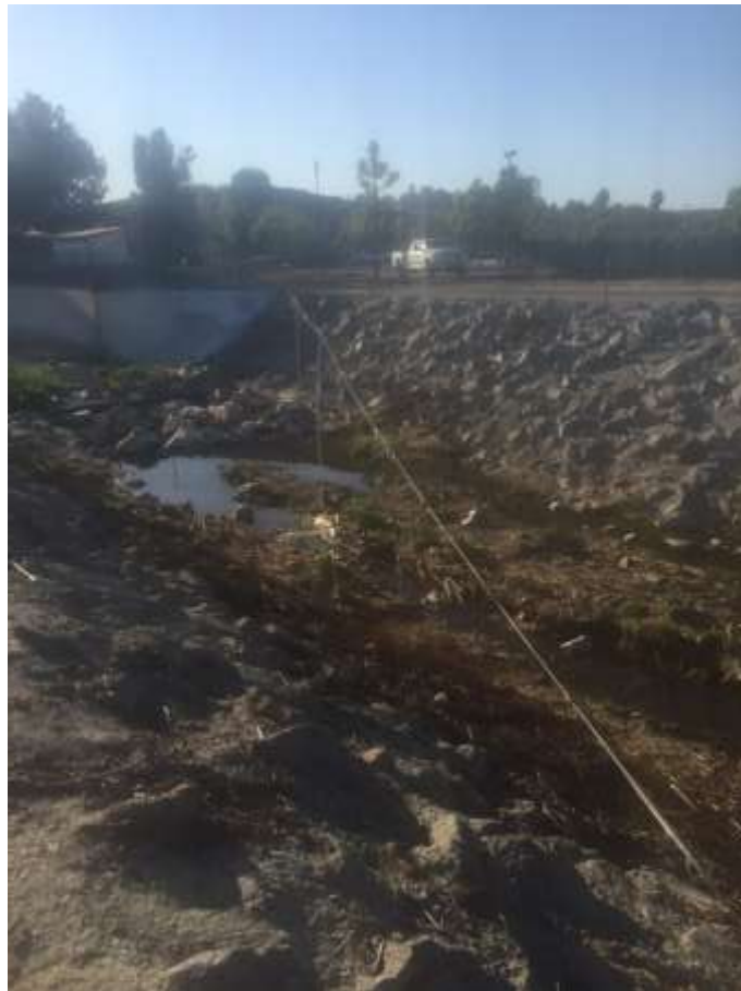
Figure 8: PVC Pipe supporting the HDD guide wire were removed from the jurisdictional drainage.
