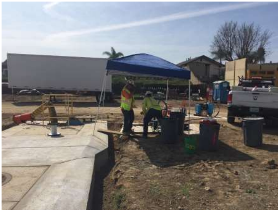
Figure 4: Conduit proofing of the HDD casings near VC #12, 500 kV Underground.
