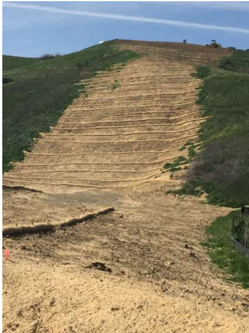
Figure 6: Permanent BMP installation between VC #3 and VC #4, 500 kV Underground.
