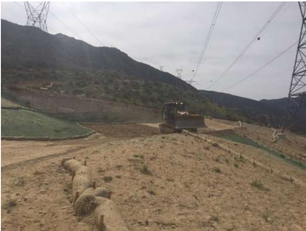
Figure 2: Decompaction and hydroseeding at Tower 54, Segment 11C.
