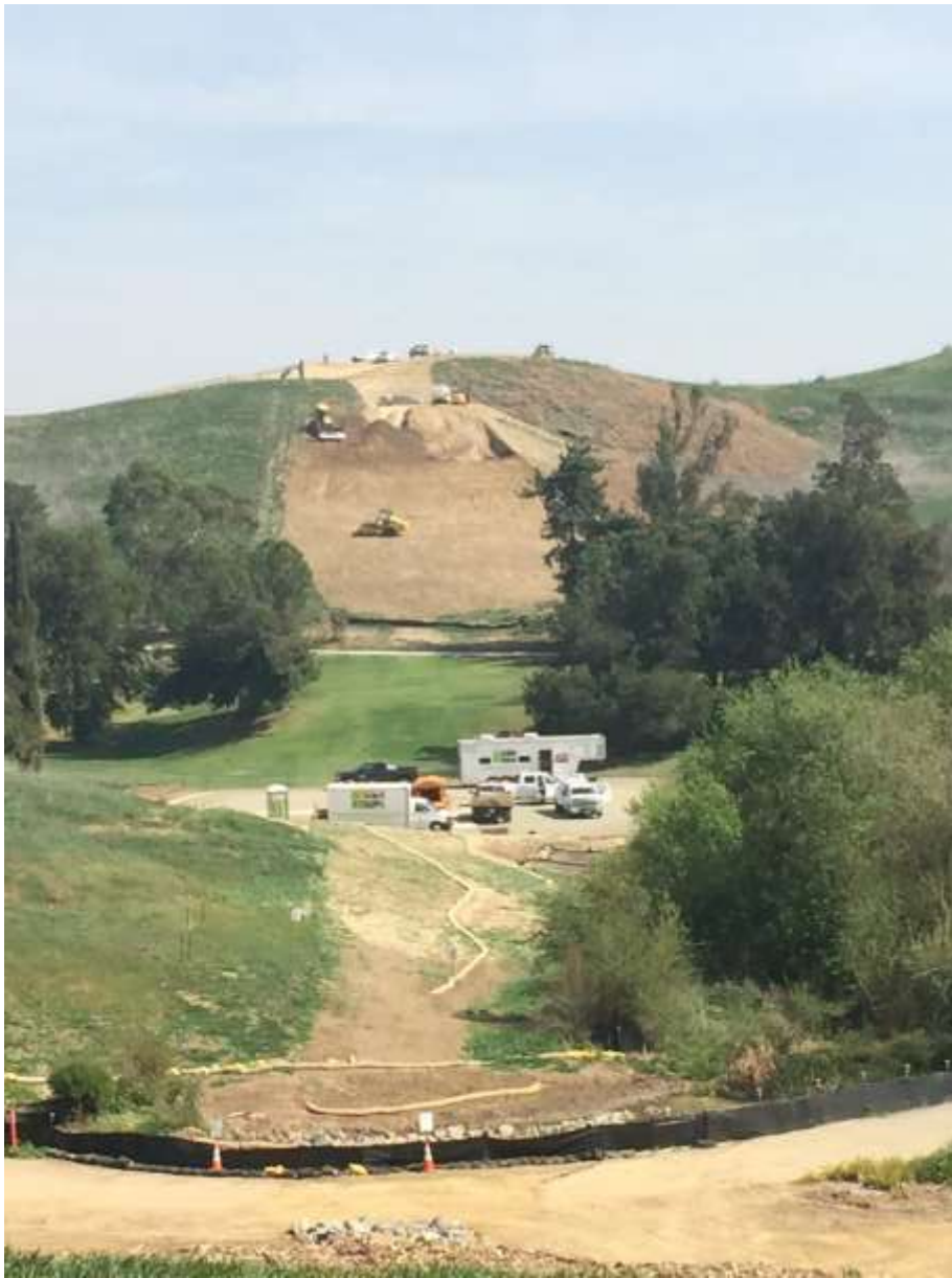
Figure 5: Restoration grading and cable splicing at VC #2, 500 kV Underground.
