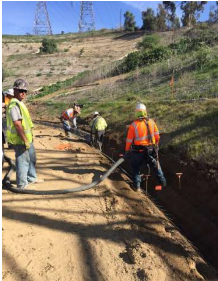
Figure 3: Concrete v-ditch installation at Tower M43-T3, Segment 8.
