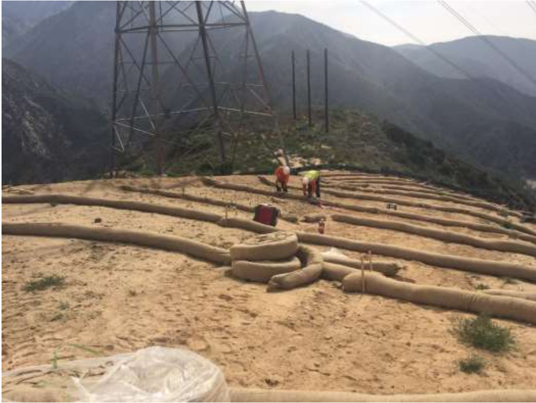
Figure 1: BMP installation after restoration grading at Tower 63, Segment 11C.
