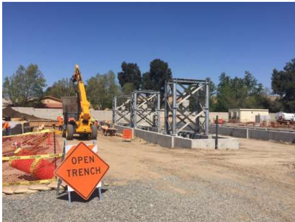
Figure 2: Construction continues at the ETS, 500 kV Underground.
