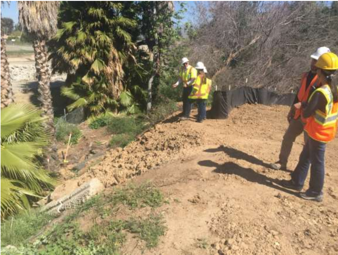
Figure 3: Site visit at the long bore location with State Water, SCE, and the CPUC EM.
