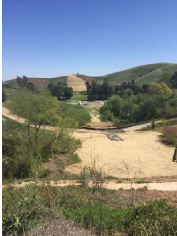
Figure 1: Stream diversion area and cable splicing at VC #2, 500 kV Underground.
