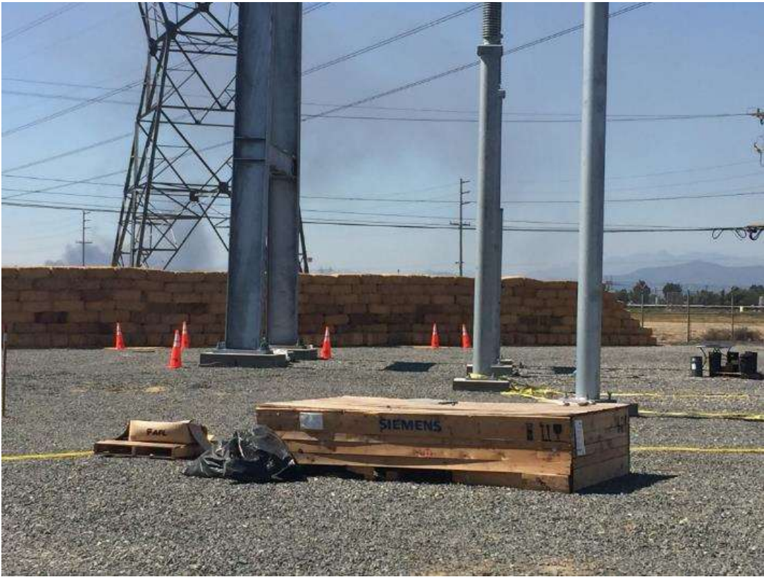
Figure 3: Sound wall constructed of hay bays along the boundary of the Mira Loma Substation, Segment 8.
