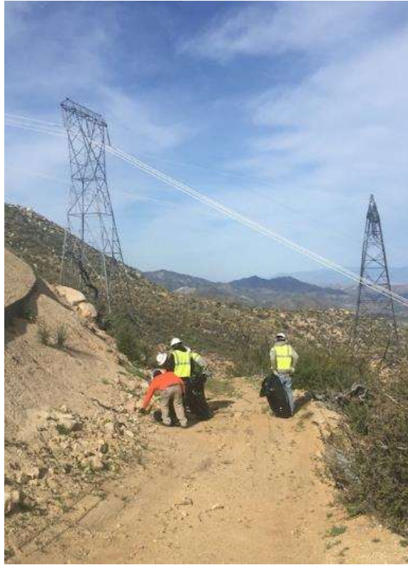
Figure 1: Weed abatement activities at Tower 20, Segment 11C. Photo courtesy of SCE.
