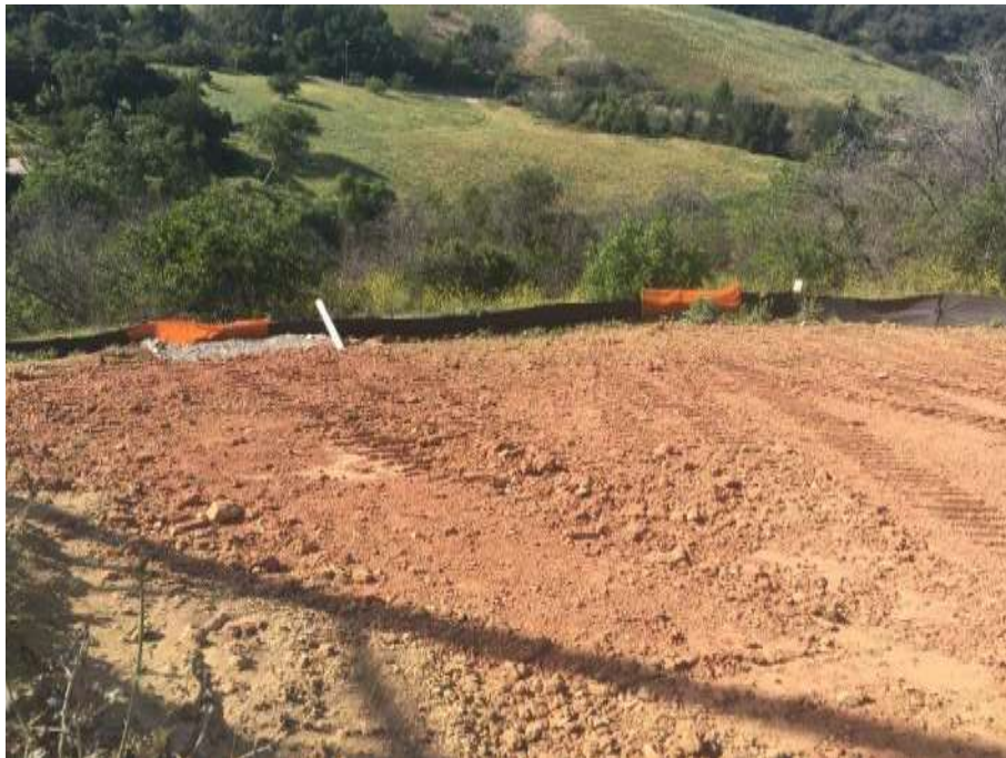
Figure 2: Civil grading work at Tower MA1-T2A, Segment 8 Phase 4.
