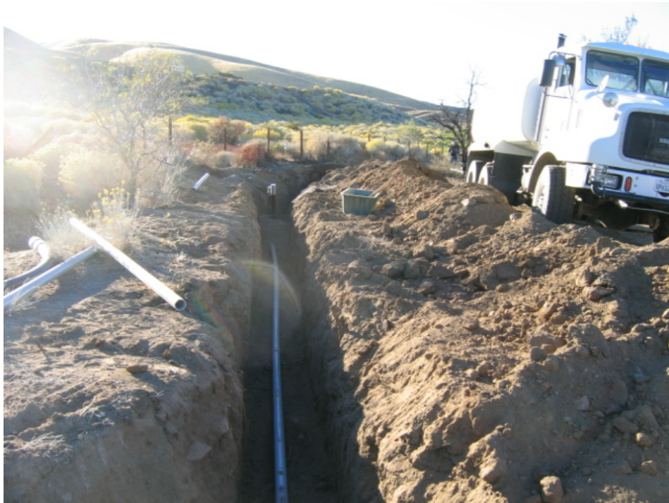
Figure 3: 12 kV underground work in Section 3.
