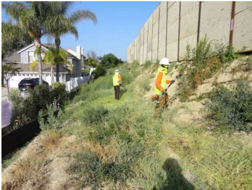
Figure 4: Vegetation management near VC #11, 500 kV Underground. Photo courtesy of SCE.
