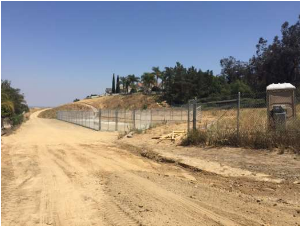
Figure 3: Partial fence installation around VC #5, 500 kV Underground.
