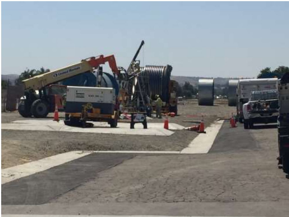
Figure 2: Cable installation operations between VC #14 and VC #13, 500 kV Underground.
