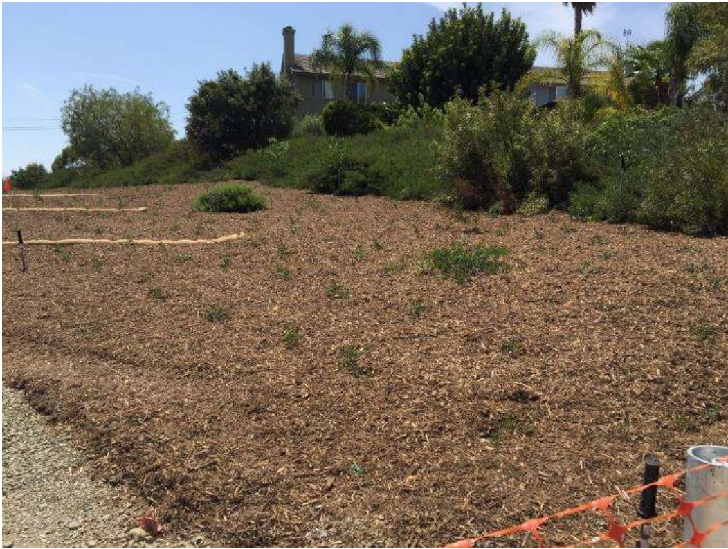
Figure 4: Landscaping crews working between VC #9 and VC #11, 500 kV Underground.
