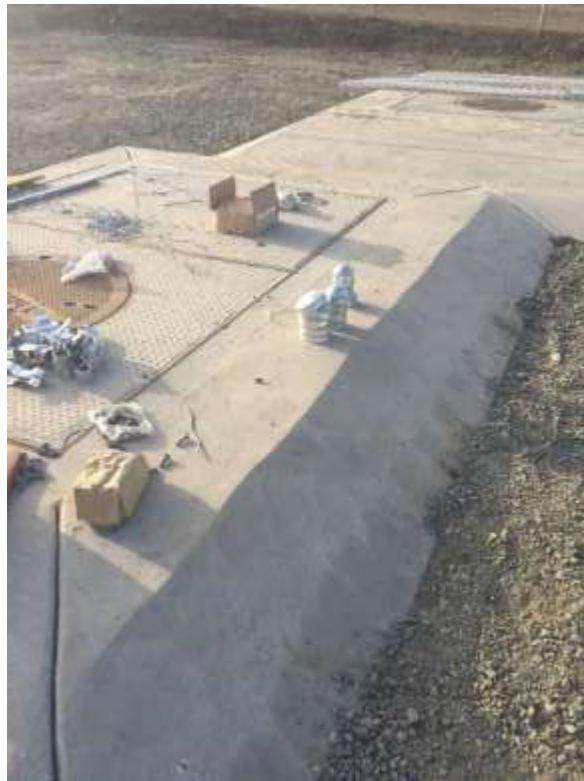
Figure 8: Fence caps were located at the vault site, 500 kV Underground.
