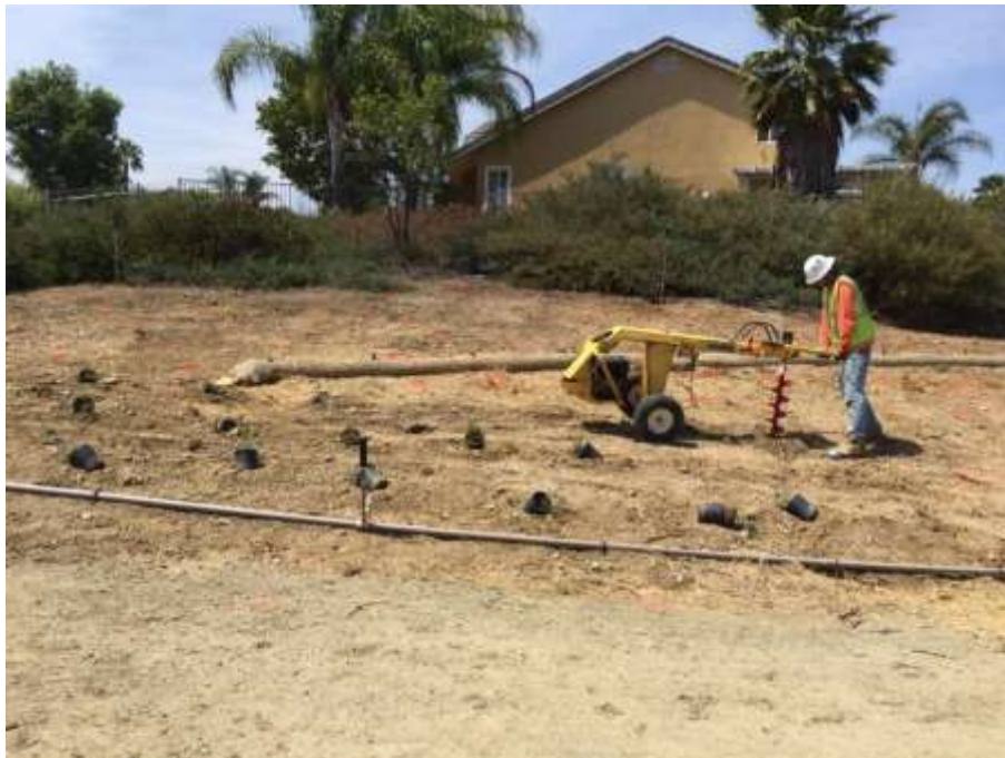
Figure 3: Landscaping crews working between VC #9 and VC #11, 500 kV Underground.
