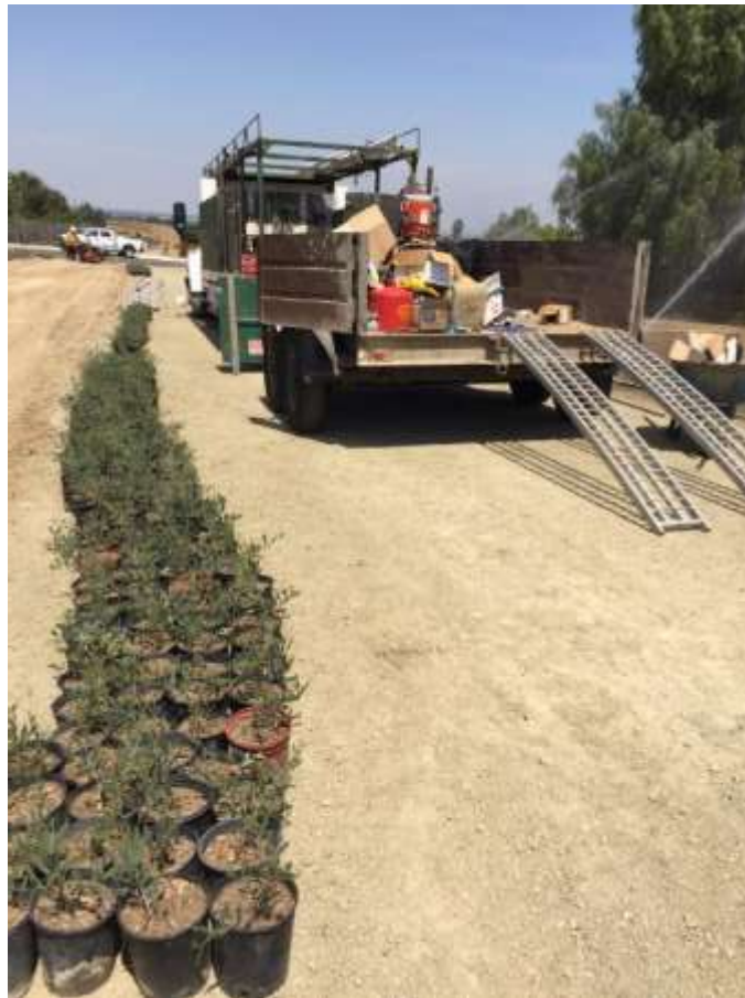
Figure 2: Landscaping crews working between VC #9 and VC #11, 500 kV Underground.
