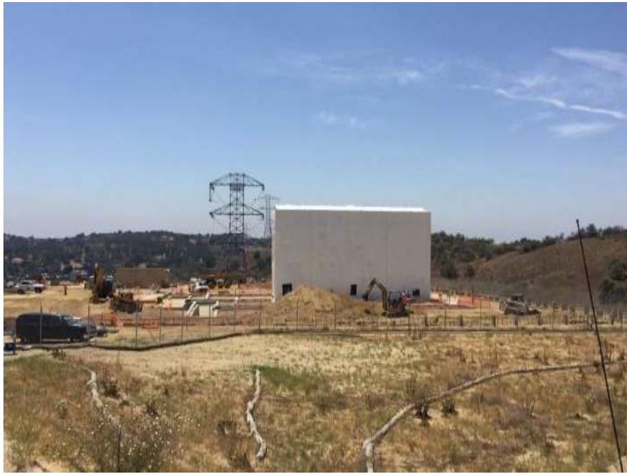
Figure 6: Work continues at the WTS, 500 kV Underground.
