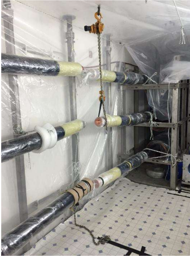
Figure 1: Splicing cable at VC #11, 500 kV Underground.
