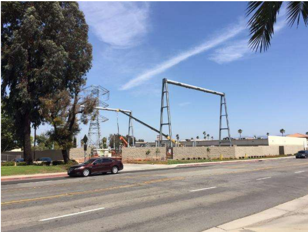
Figure 5: Dead end bus structure installation at the ETS, 500 kV Underground.
