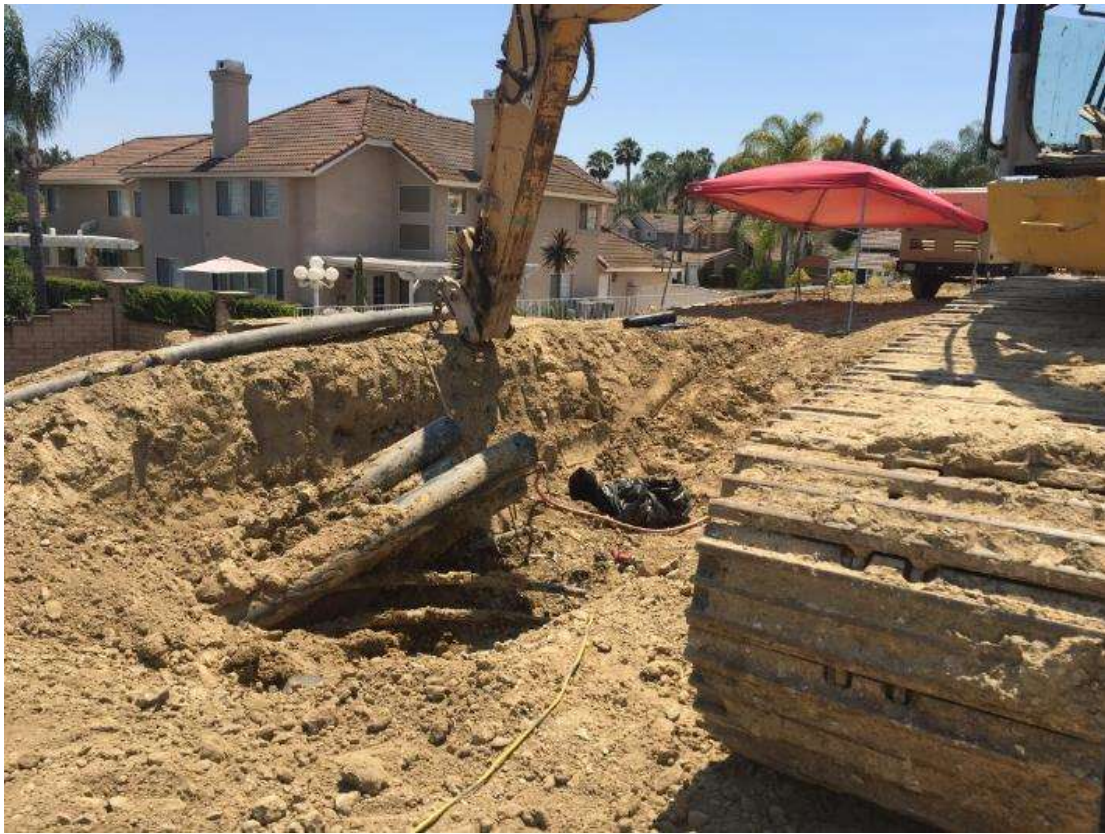
Figure 3: HDD casing was successfully pulled back on June 20, 500 kV Underground.
