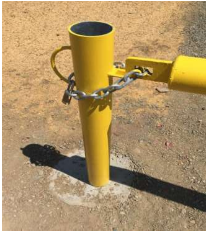
Figure 5: Open pipe gate post near Restraint Vault #4, 500 kV Underground. SCE has since capped the open pipes.
