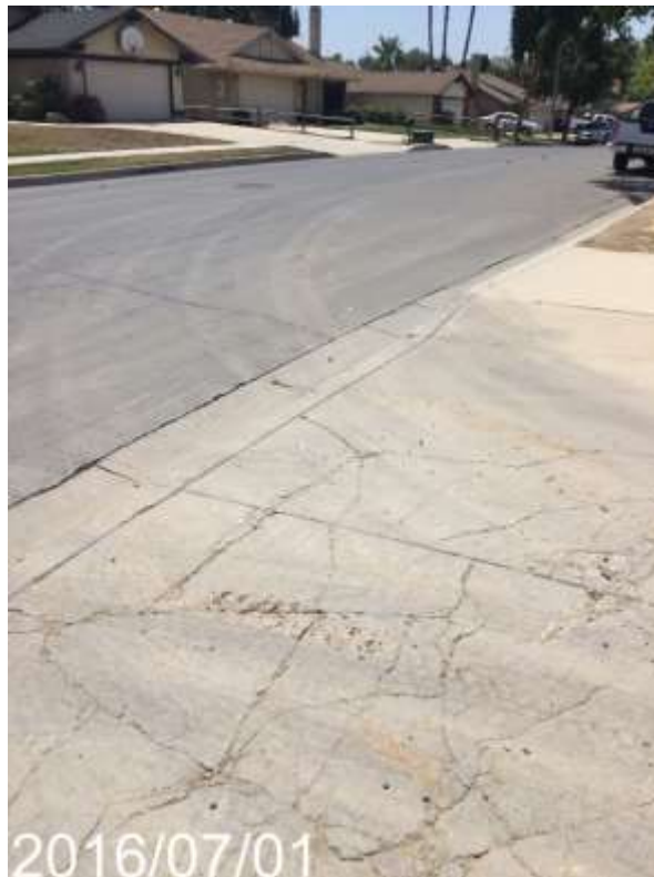
Figure 2: Trackout reported along Cork Drive, 500 kV Underground. Photo courtesy of SCE.
