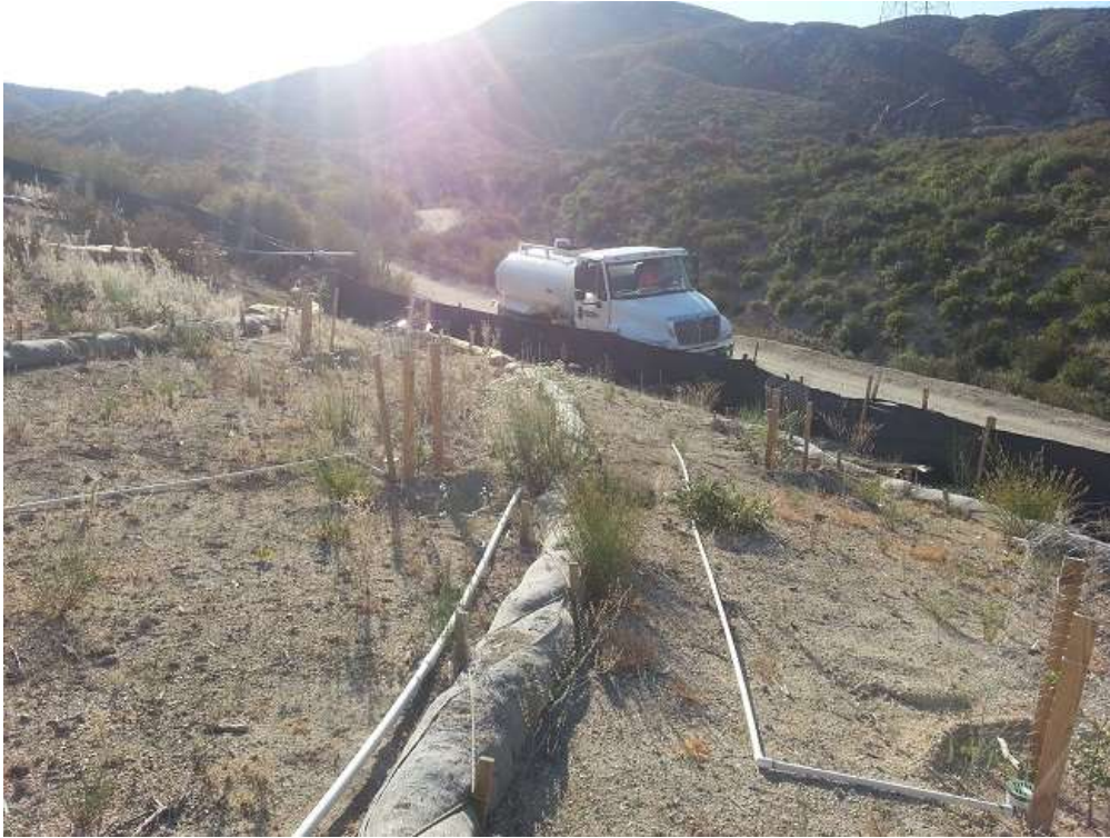
Figure 1: Irrigation system installation at Pullsite 62/63 on Segment 6. Photo courtesy of SCE.
