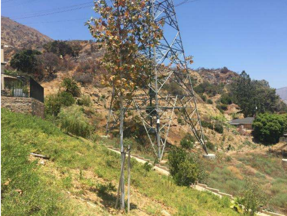
Figure 1: The recent fire damage at Tower M27-T2 damaged the irrigation system installation already in place, Segment 7.
