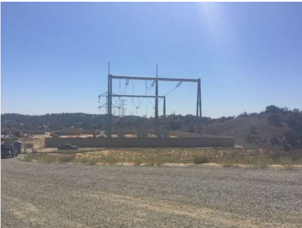
Figure 4: The recently completed block wall at the WTS, 500 kV Underground.
