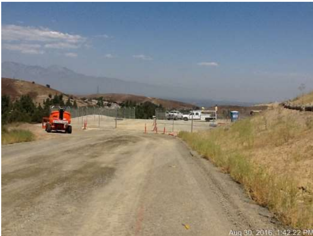
Figure 2: Vault cluster fencing installation continued at VC #1.
