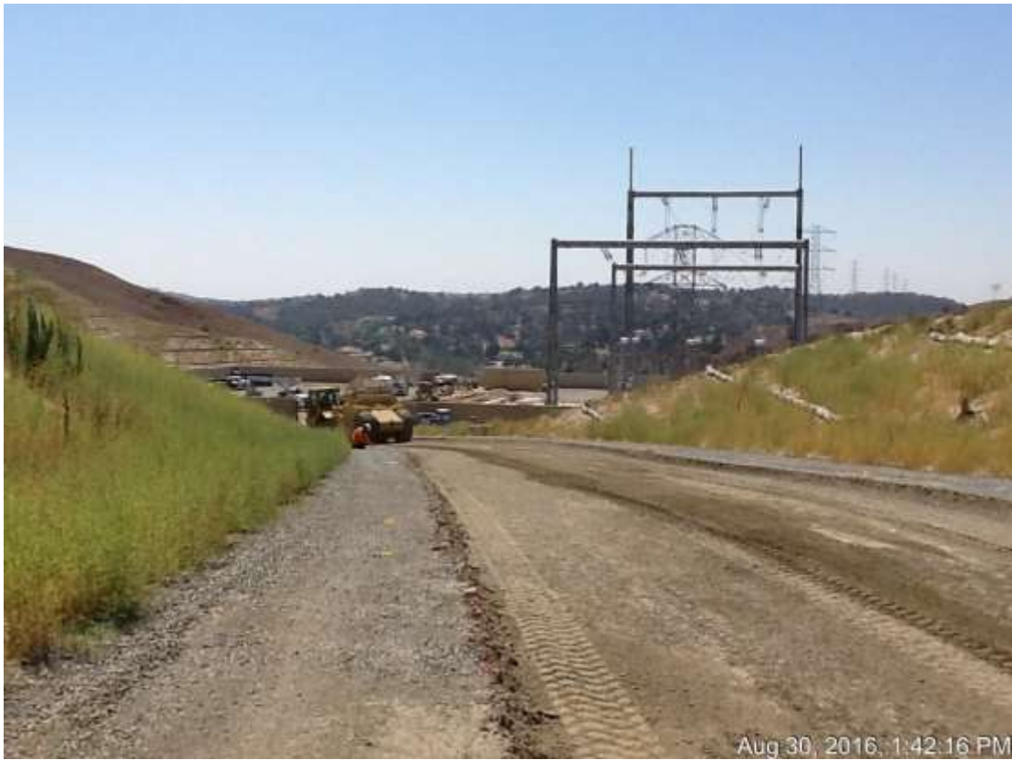
Figure 3: Road base installation on the WTS access road, 500 kV Underground.
