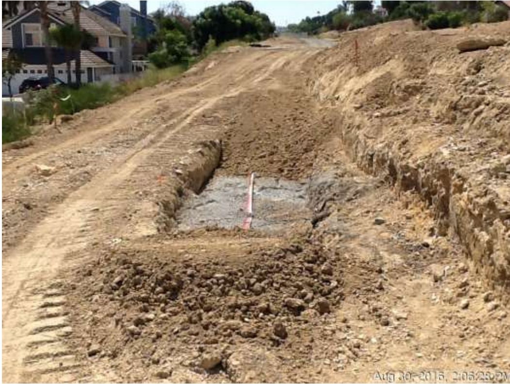
Figure 1: Tie ins and burial of the HDD casings near VC #11.
