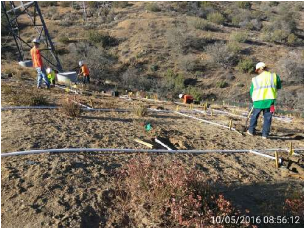
Figure 2: Container plant installation at Tower 2, Segment 11. (Photo courtesy of SCE.)
