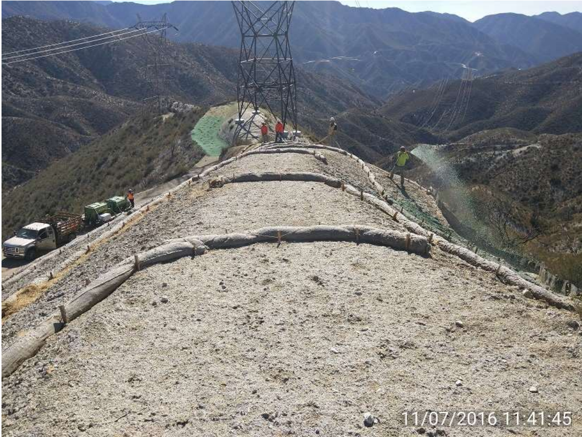
Figure 1: Hydroseeding at Restoration Site 35, Segment 11. (Photo courtesy of SCE.)
