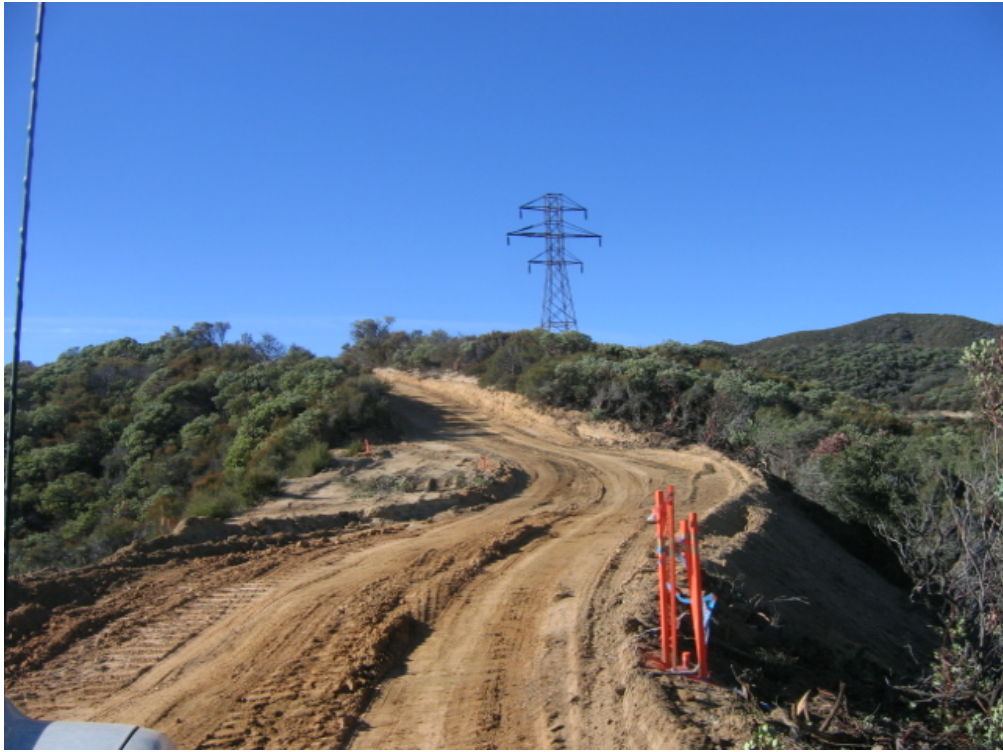
Figure 2: Widening of ANF road to avoid tower 88 foundation.
