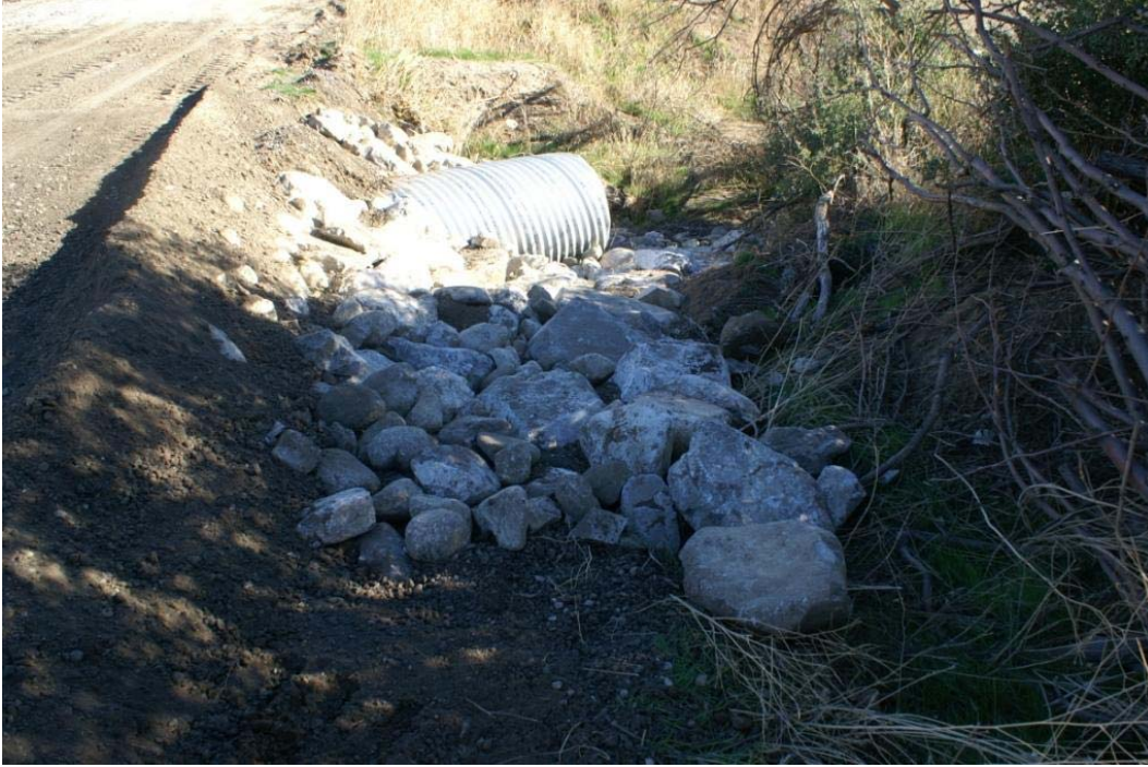
Figure 1: Blue Cloud road culvert improvement with riprap.
