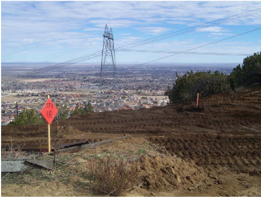
Figure 3: Crane pad construction at Tower 18, Segment 2.
