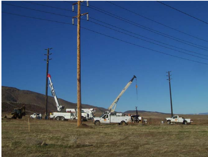
Figure 2: 66 kV pole relocation, Segment 2.
