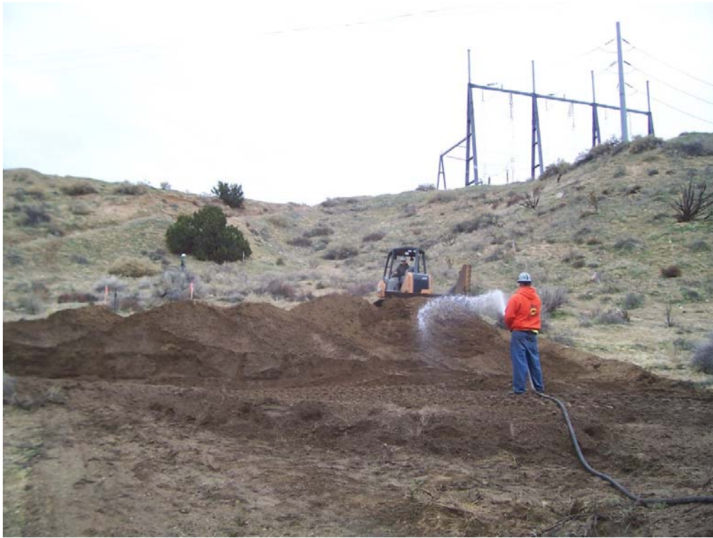
Figure 2: Site preparation of Tower 120, Segment 2.
