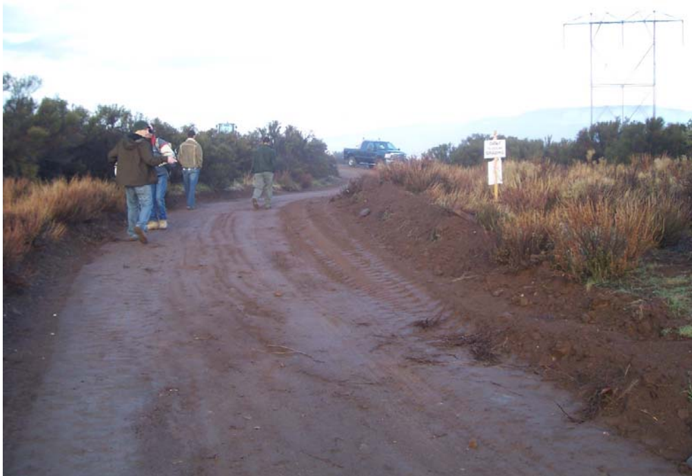
Figure 3: Heavy equipment tracks after ground disturbance within ESA, Segment 2.
