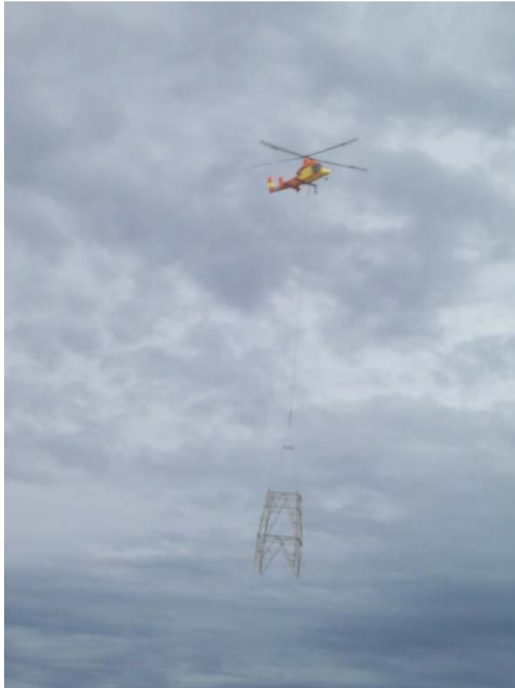
Figure 1: 66 kV tower removals in Section 2, Segment 1 on the ANF.
