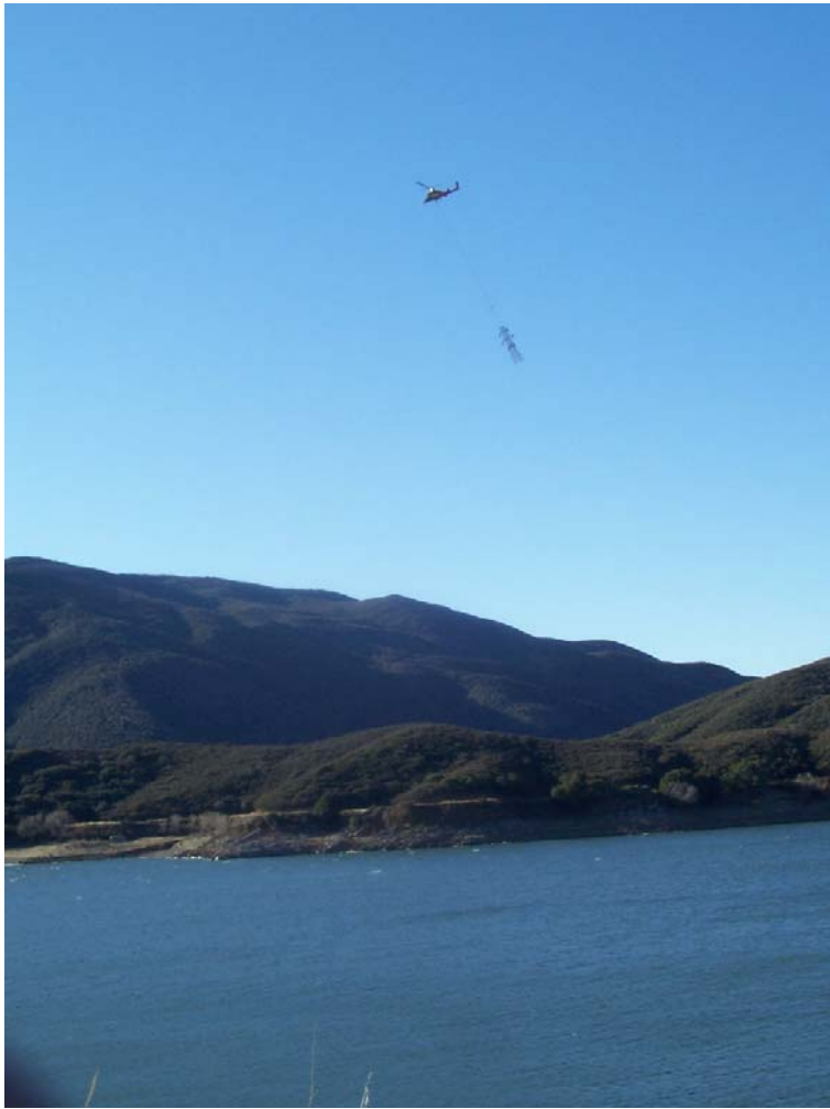
Figure 2: 66 kV tower removal on the ANF.
