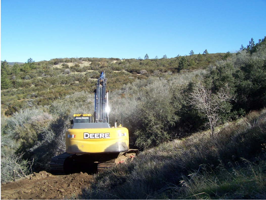
Figure 1: Spur Road 73 construction on the ANF, Segment 1, Section 2.
