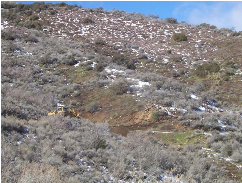
Figure 2: Access road improvement between Towers 58-64, Segment 2.
