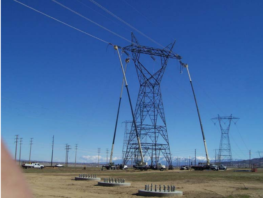
Figure 1: Lift structure M88-T1A has been completed, Segment 1, Section 3.
