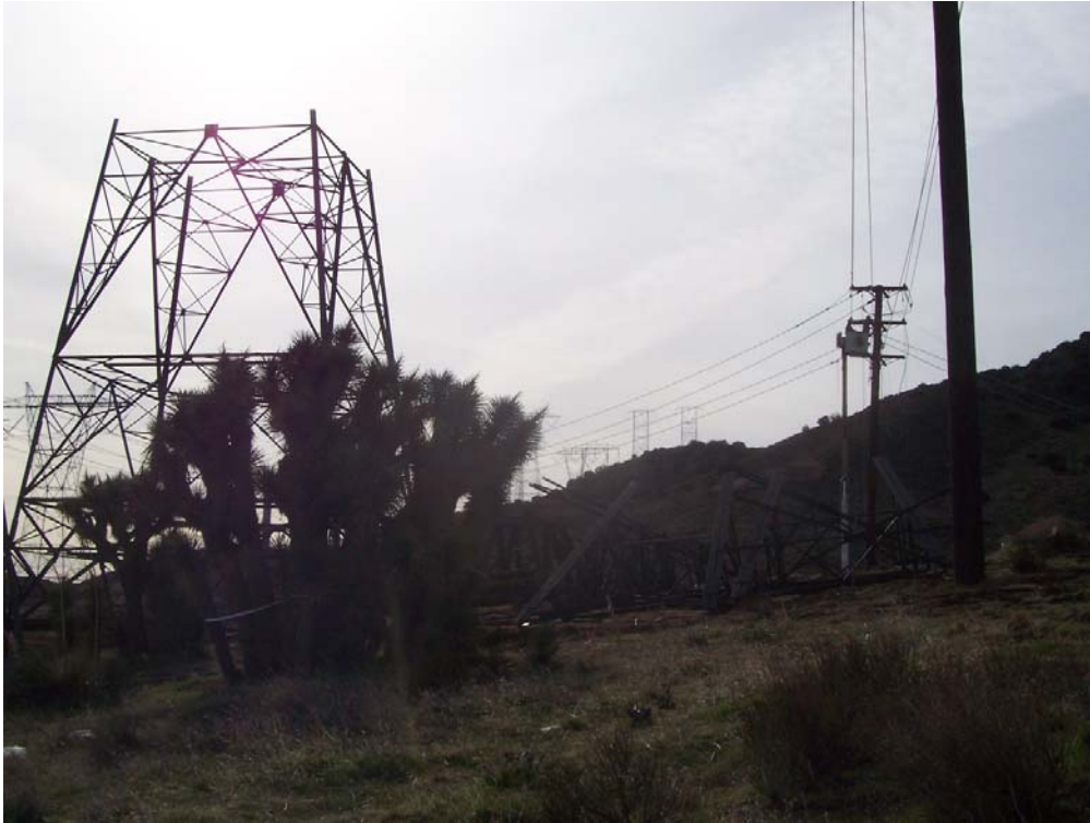
Figure 1: Steel assembly at Tower 17 and 66 kV pole installation and removal, Segment 2.
