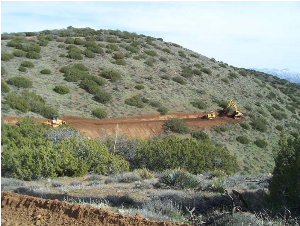
Figure 2: Road building near Tower 90 in Segment 2.
