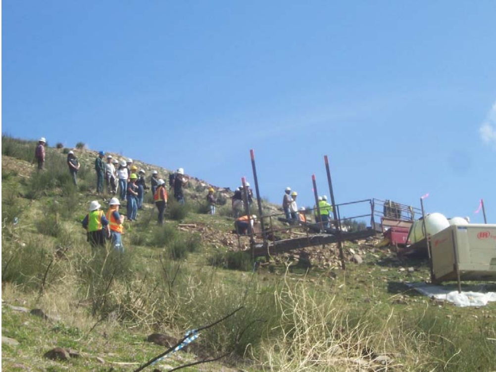
Figure 1: Micropile foundation demonstration at Tower 54 in Section 2, ANF.
