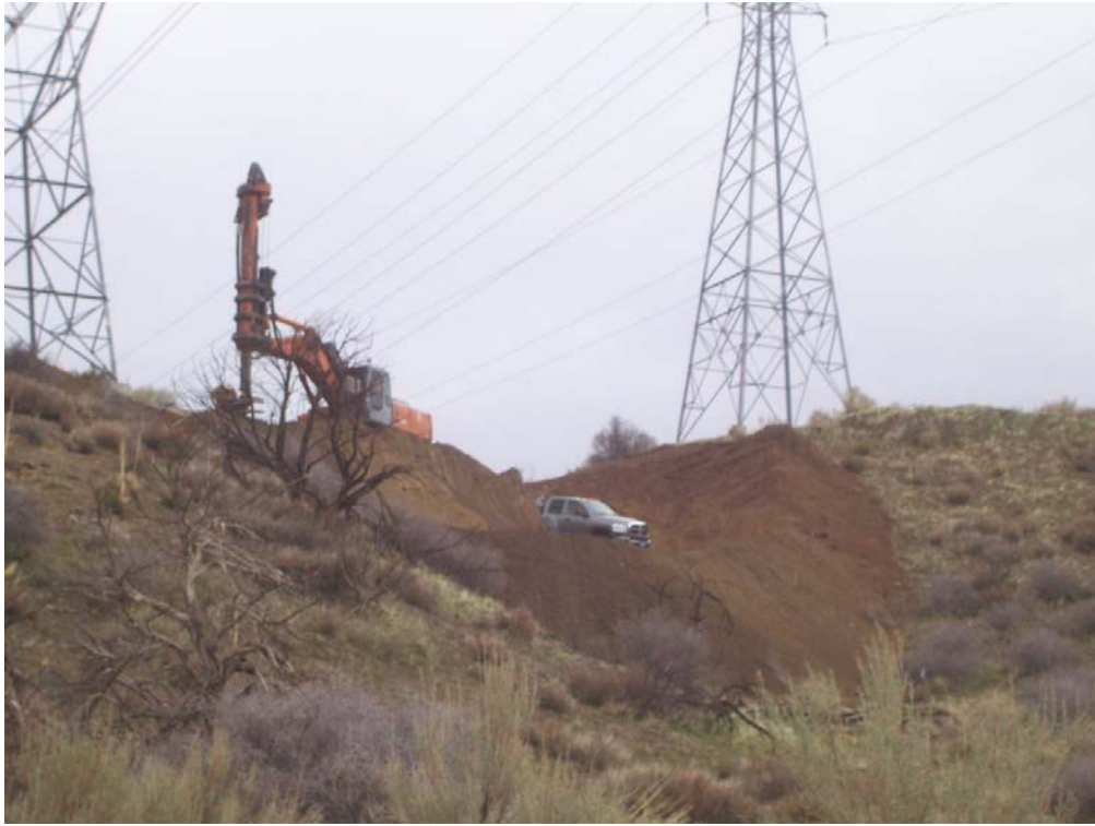
Figure 3: Foundation drilling at Tower 22, Segment 2.
