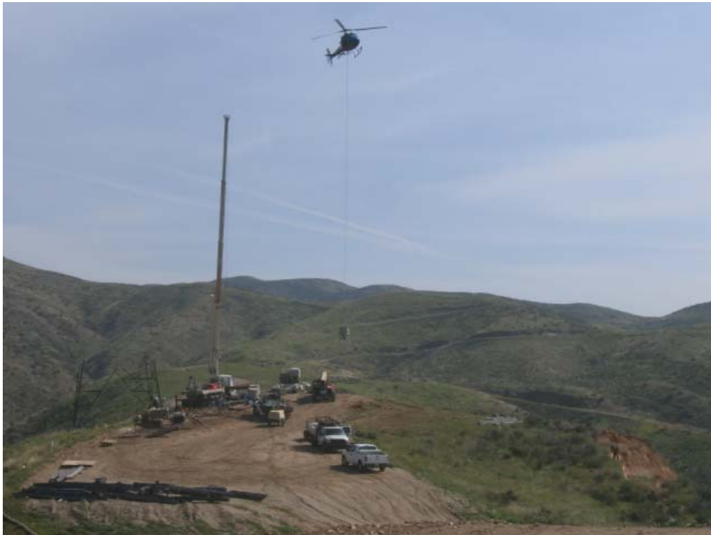
Figure 4: Grout preparation and helicopter delivery in the ANF, Section 2.
