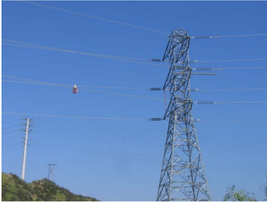
Figure 1: Spacer installation between Towers 1b and 2 in Santa Clarita.
