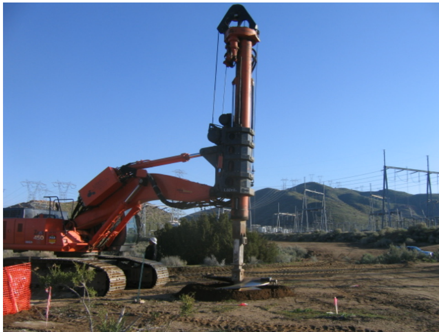
Figure 6: Foundation drilling near the Vincent Substation.
