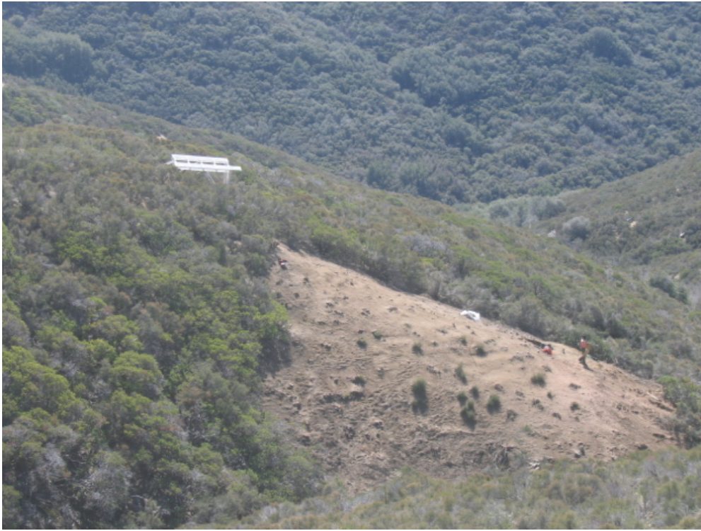
Figure 3: Cleared tower pad in the ANF, Section 2.
