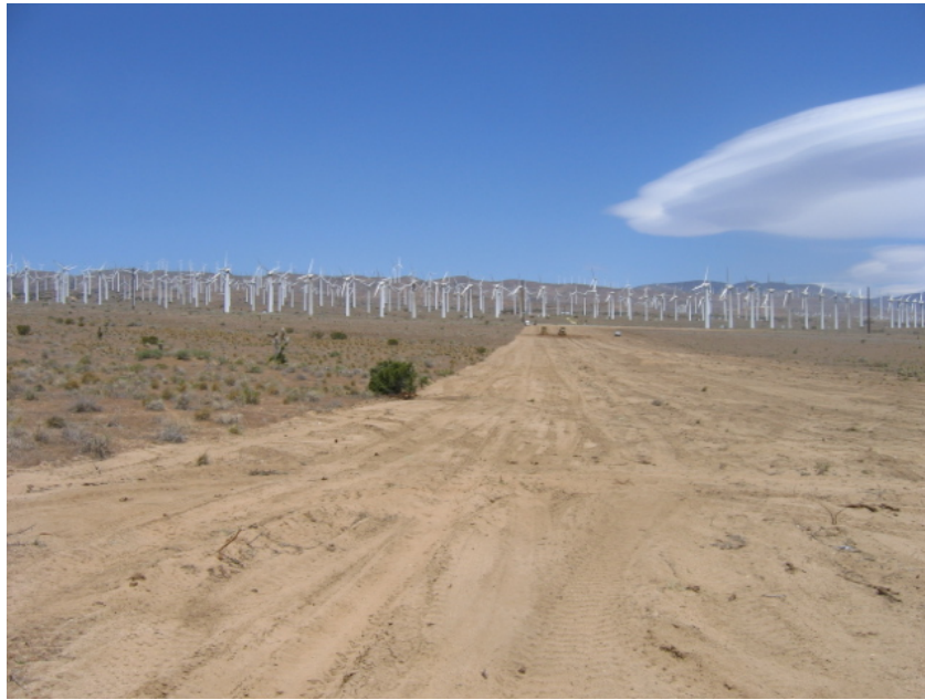
Figure 3: Grading and brush clearing of the new Windhub Substation.
