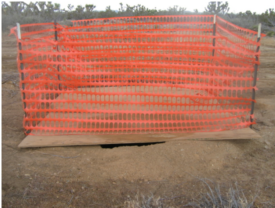
Figure 2: Gaps between the ground surface and plywood covers in desert tortoise areas of Segment 3A.
