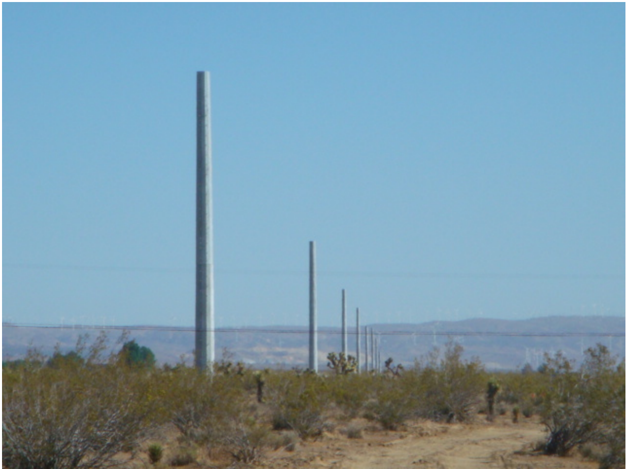
Figure 4: Tubular Steel Pole (TSP) bases in place in Segment 3A
