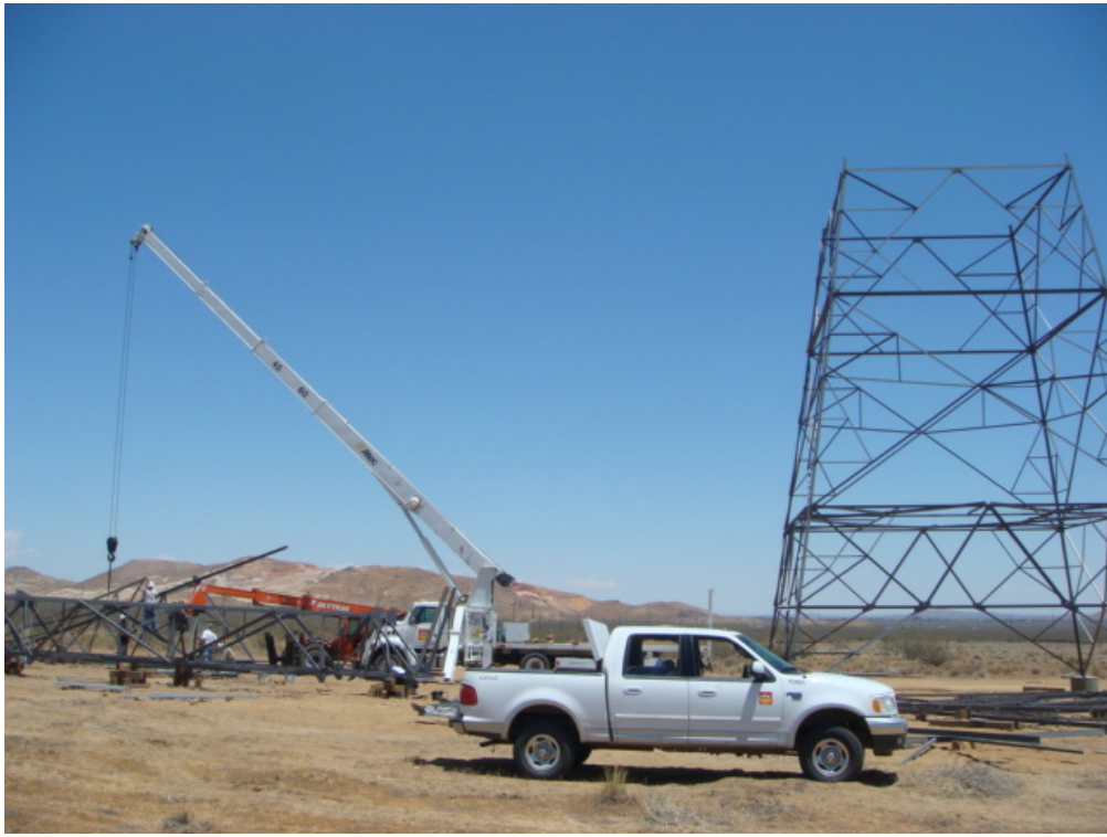
Figure 4: Assembly of lattice steel towers at Structure 25, Segment 3A.
