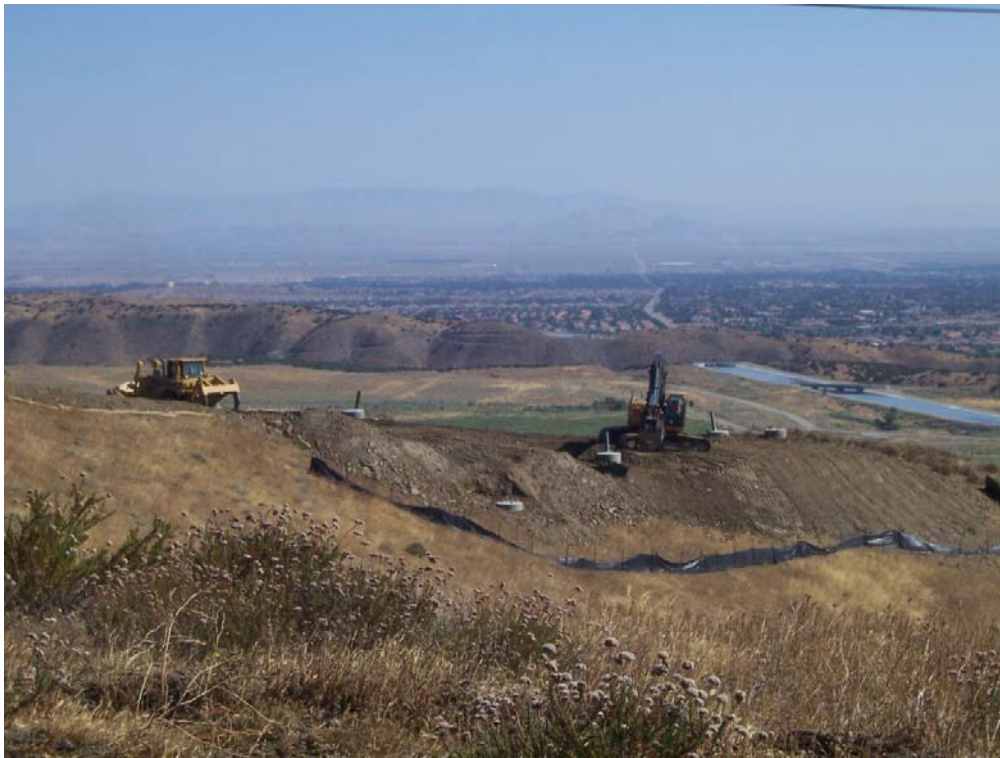
Figure 3: Foundation reveals and crane pad extension prior to tower assembly, Segment 2.
