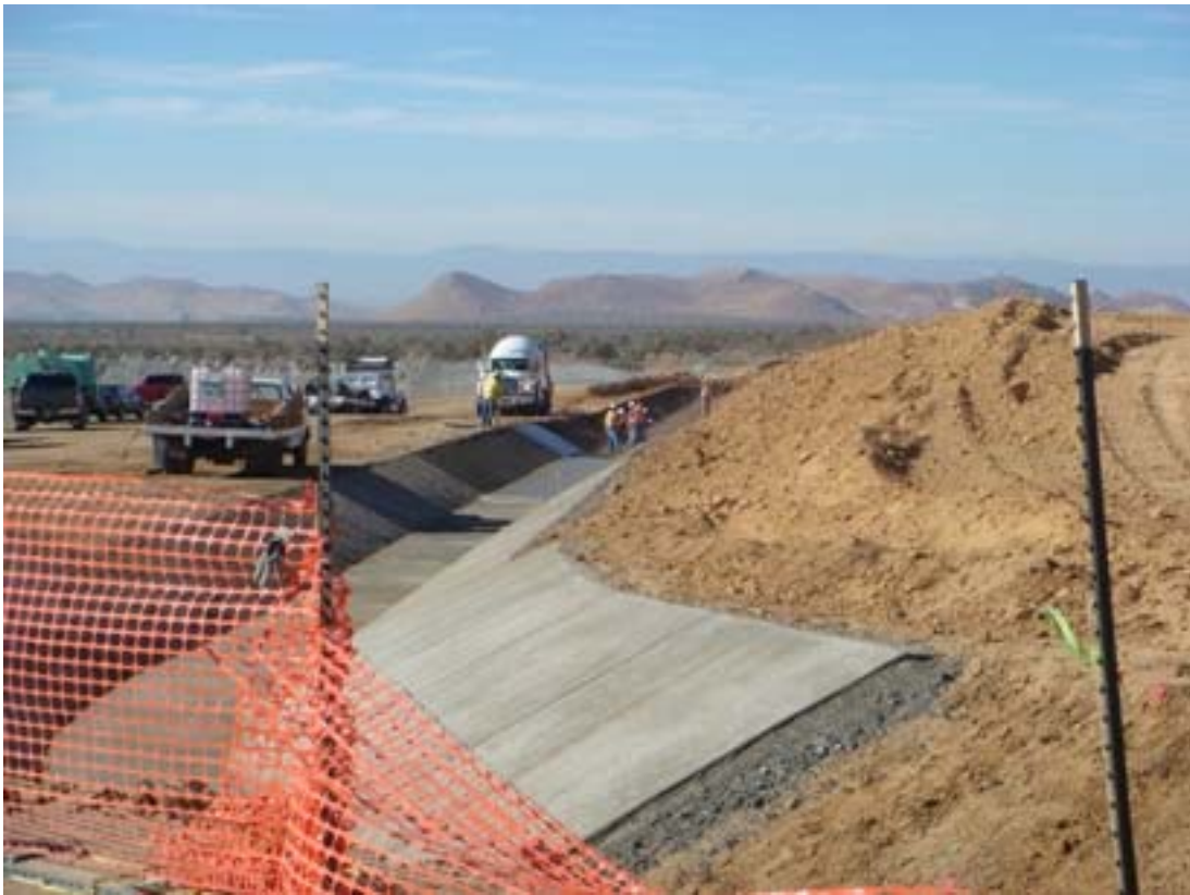
Figure 3: Concrete drainage channel at the Windhub Substation.
