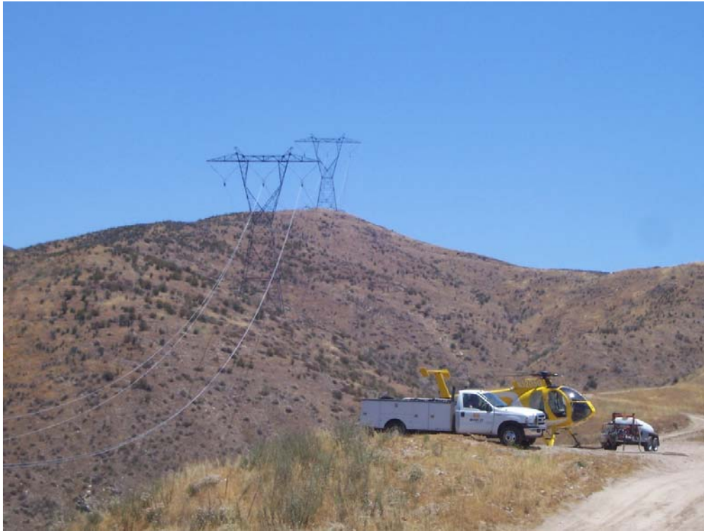
Figure 1: Wire stringing between Towers 33 and 41 Segment 1, Section 2.
