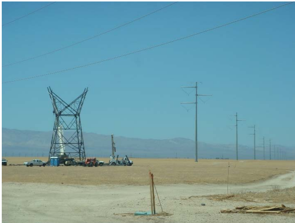
Figure 2: Assembly of lattice steel towers at Structure 95, Segment 3A.
