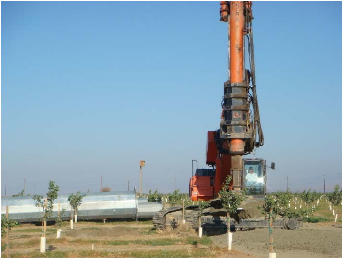
Figure 4: Foundation drilling at Tower 60, Segment 3A.
