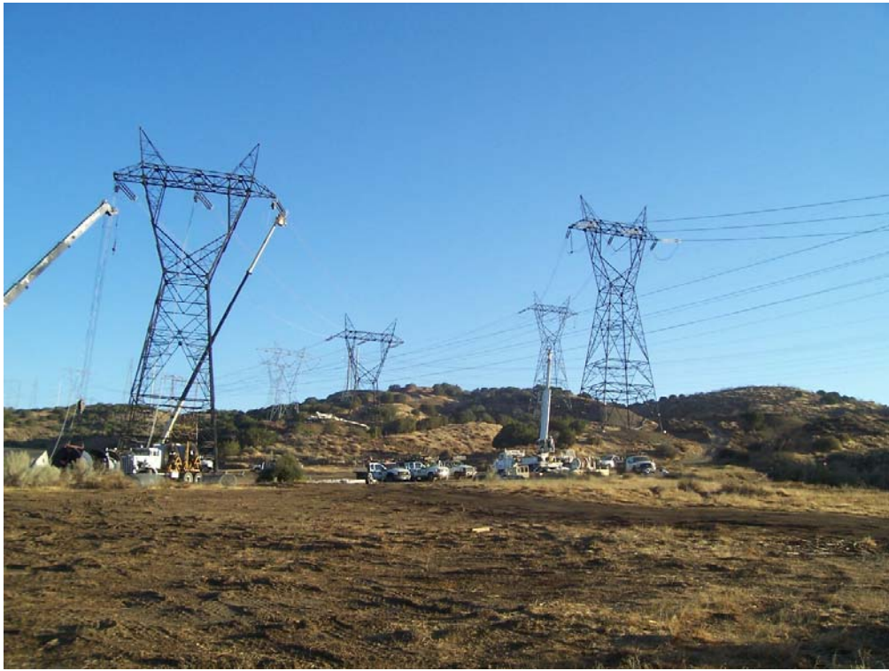
Figure 3: Wire stringing between Towers 33 and 35, Segment 2.
