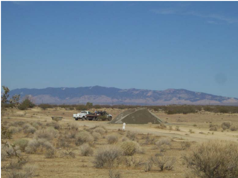
Figure 4: Stockpiling of capping materials, Segment 3A.
