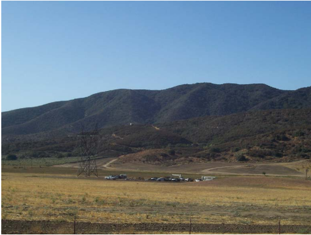
Figure 1: Last section of wire stringing installation on Segment 1, Section 3.
