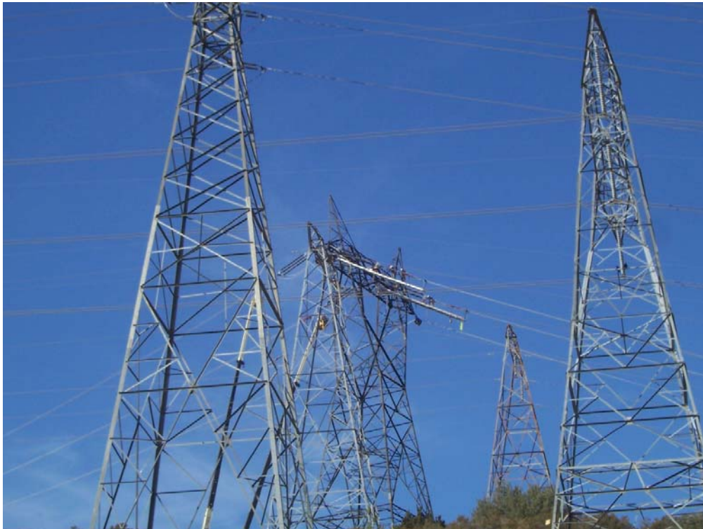
Figure 2: Conductor installation between Towers 36 to 39, Segment 2.
