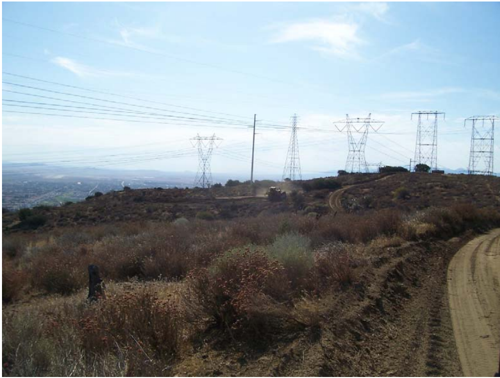
Figure 3: Recontouring at Tower 23, Segment 2.
