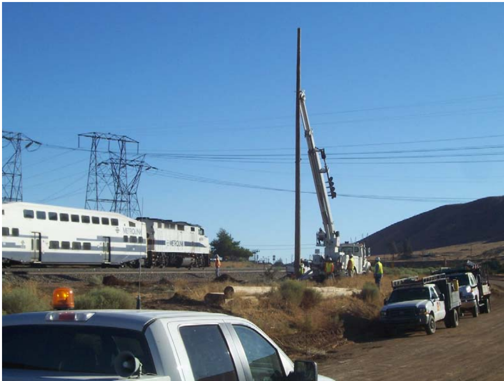
Figure 2: Guard pole installation Segment 2, crossing the Metrolink tracks.
