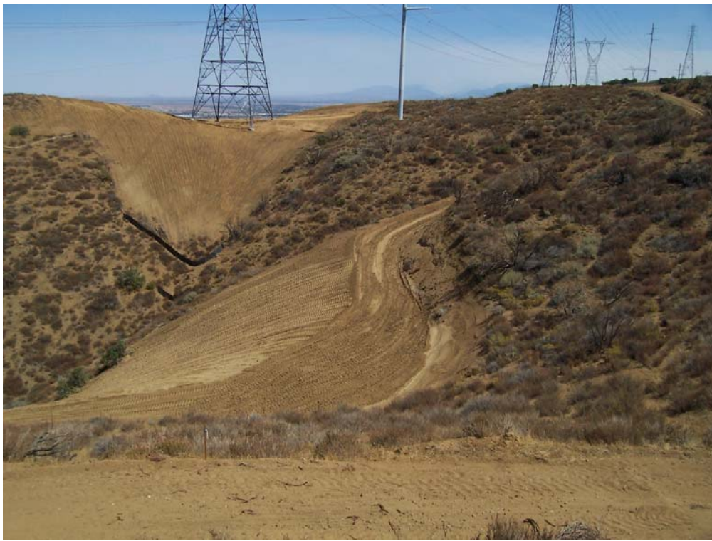
Figure 3: Recontouring at Tower 23, Segment 2.
