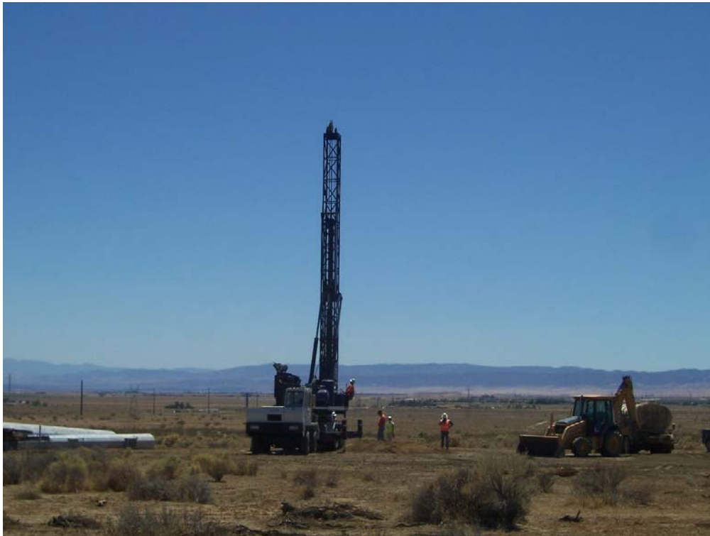
Figure 4: Drilling Tower 44, Segment 3A.
