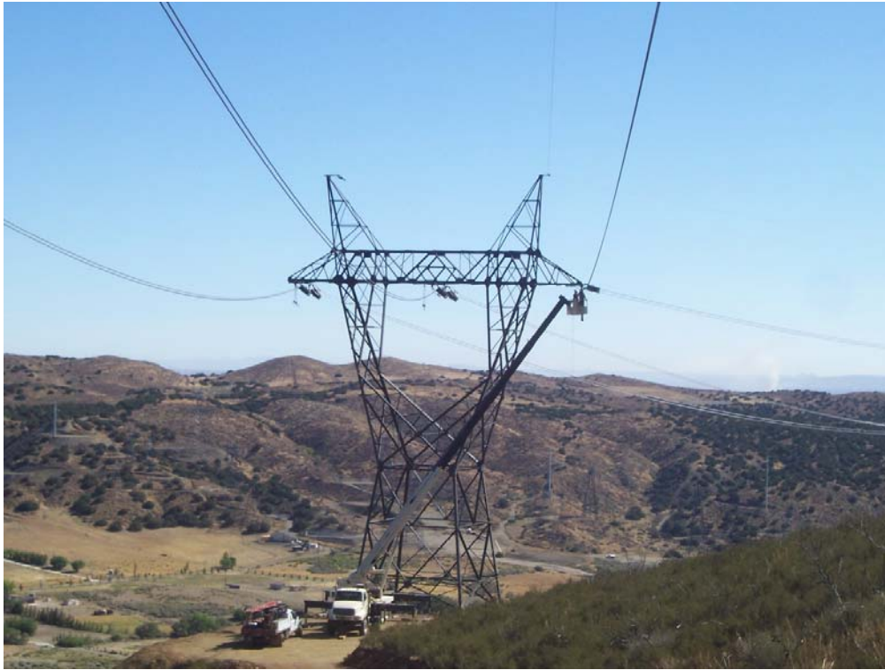
Figure 1: Wire stringing installation on Segment 2 between Towers 39-51.
