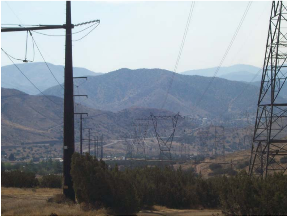
Figure 1: Wire stringing installation on Segment 2 between Towers 105-113.
