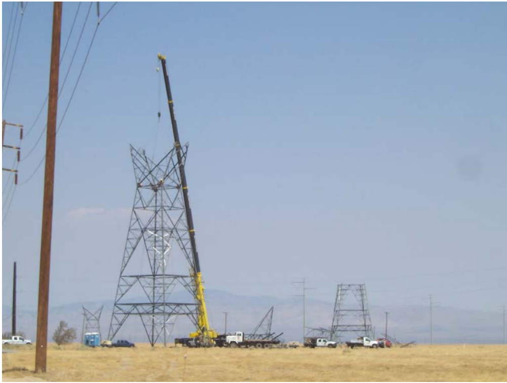
Figure 3: Lattice tower steel assembly Segment 3.
