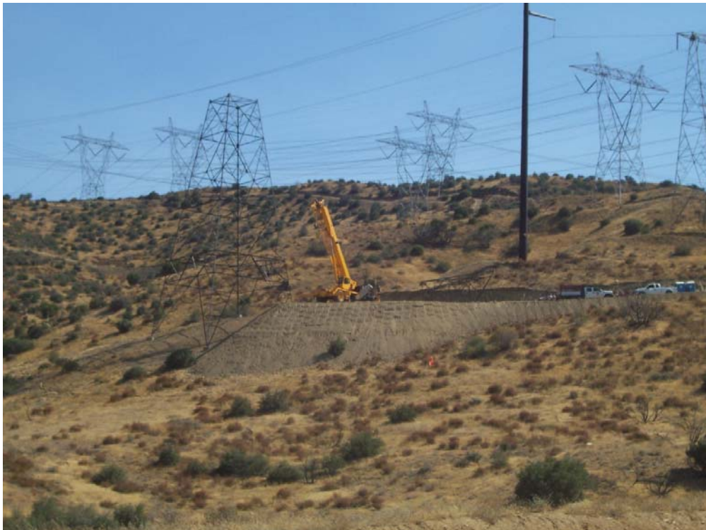
Figure 2: Lattice tower steel assembly Segment 2.
