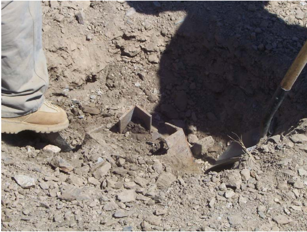
Figure 1: 66 kV lattice tower footing excavation and removal on the ANF.
