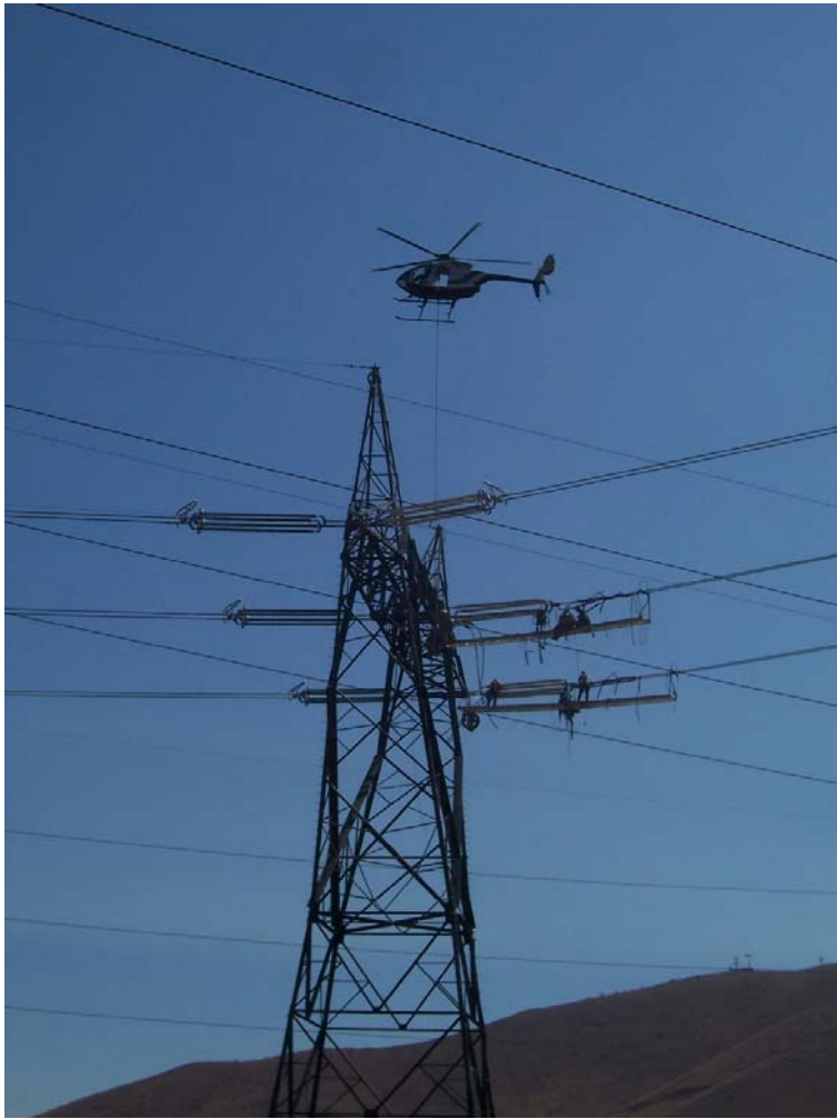
Figure 3: Wire stringing between Towers 110-113 Segment 2.
