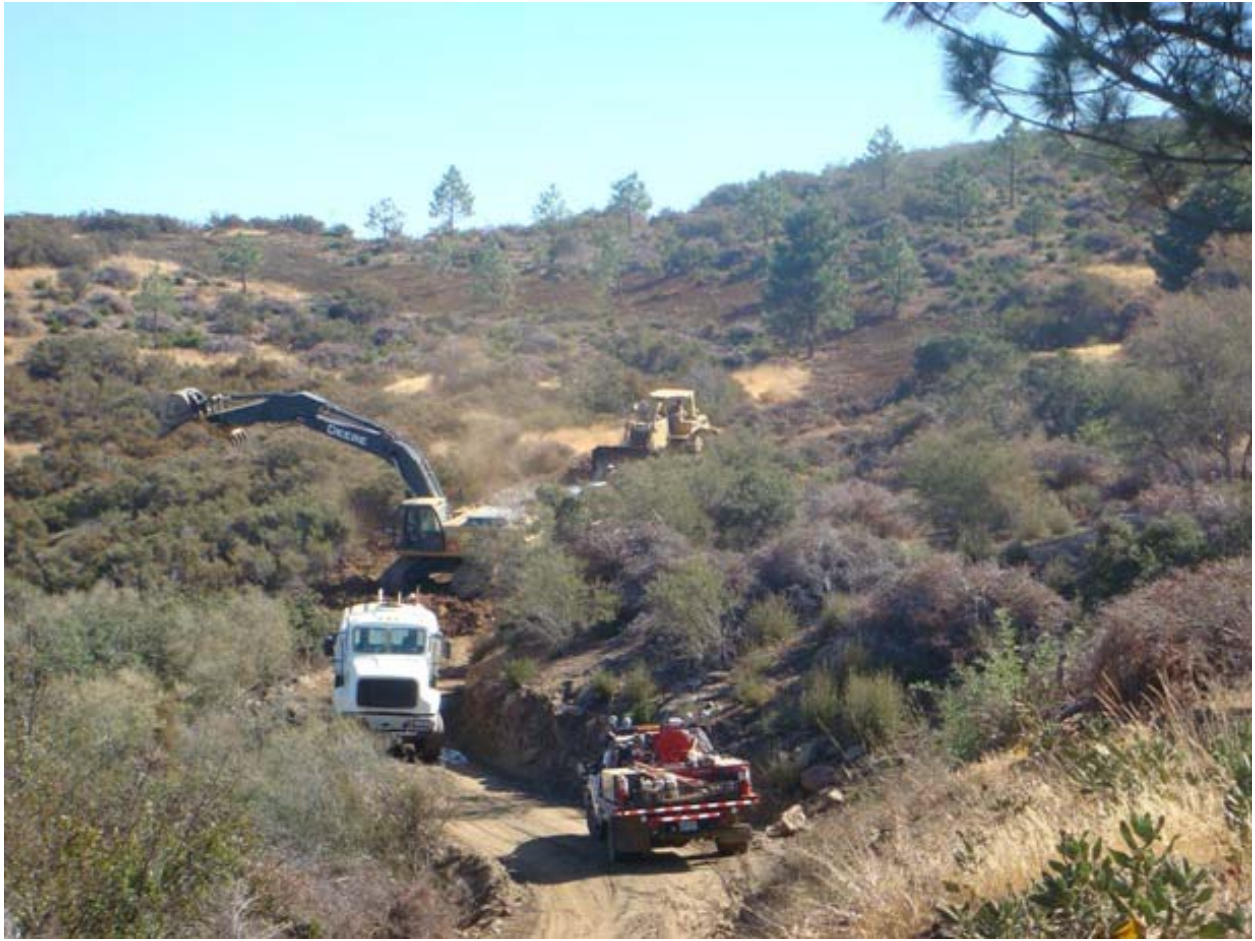
Figure 1: Recontouring of Spur Road 73 on the ANF.
