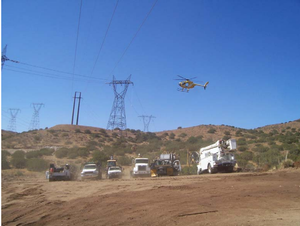
Figure 4: Wire stringing between Towers 95-105, Segment 2.
