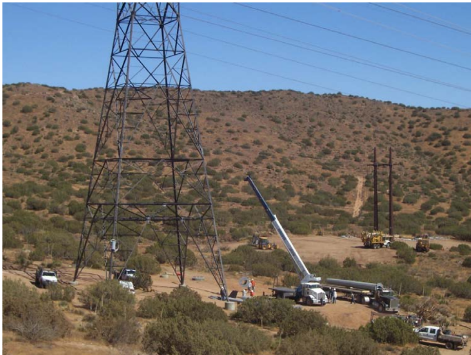
Figure 3: Transposition steel pole delivery to Tower 106, Segment 2.
